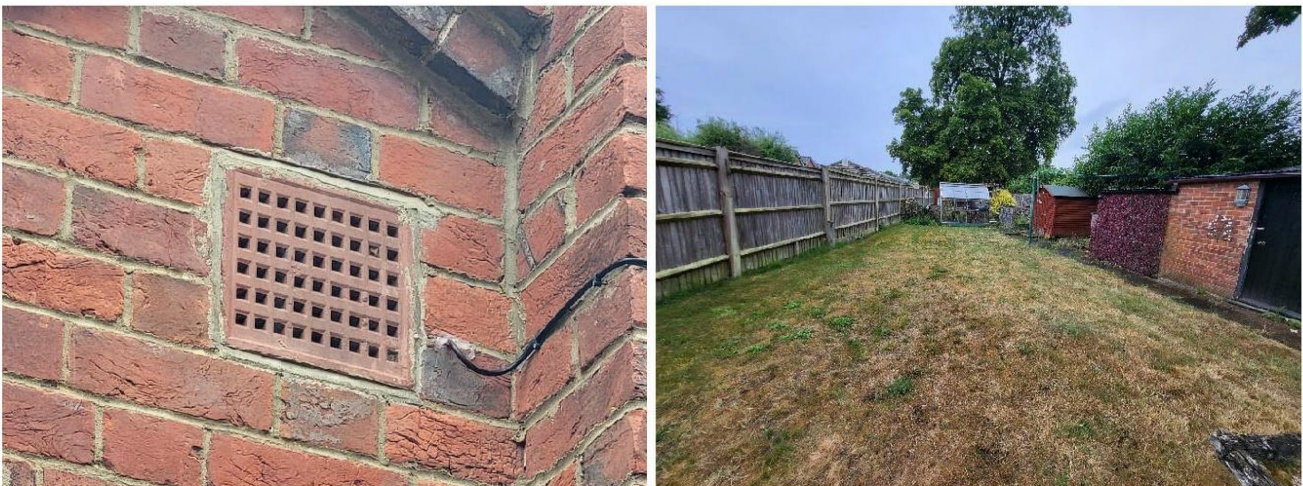
Figure 9. View of the ventilation grill (left) - View of the garden (right)
