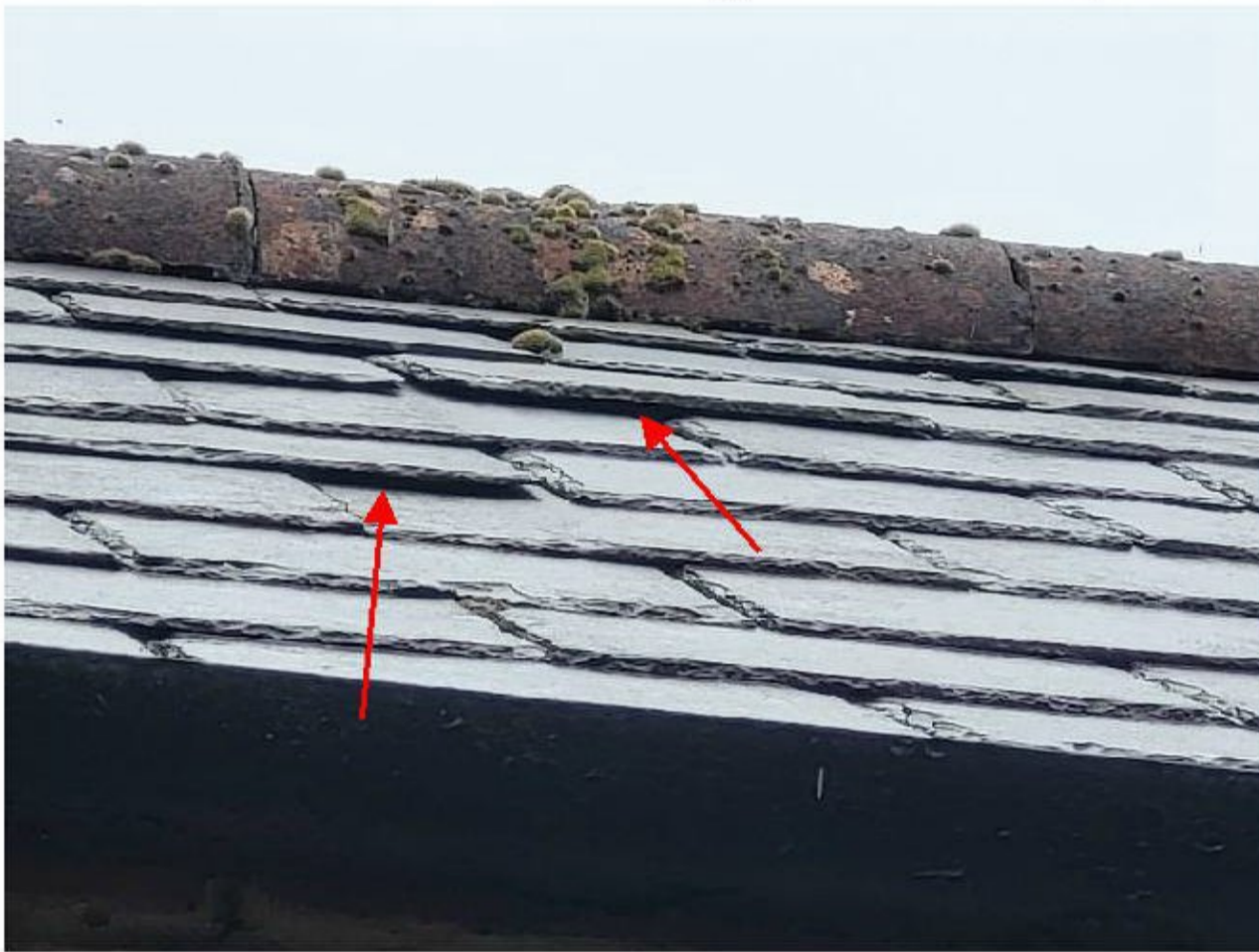
Figure 5. Example of slightly lifted roof slates
