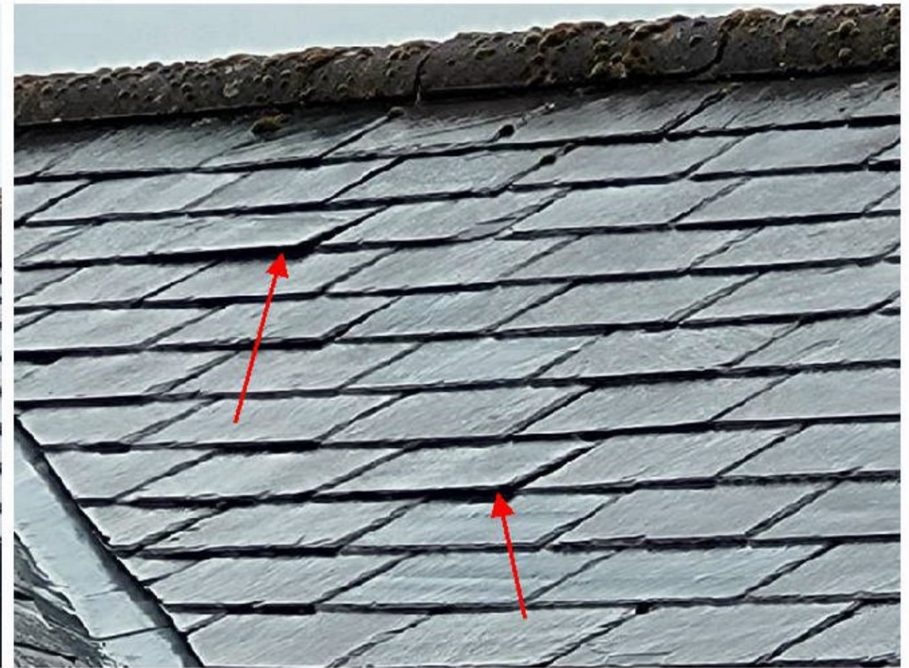
Figure 5. Example of slightly lifted roof slates
