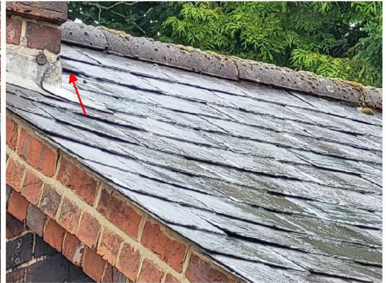
Figure 6. Example of slightly lifted roof slates
