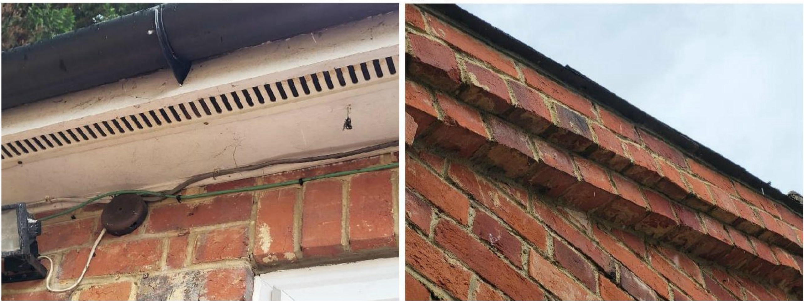
Figure 8. Example of tightly fitted soffit and the well-sealed eaves
