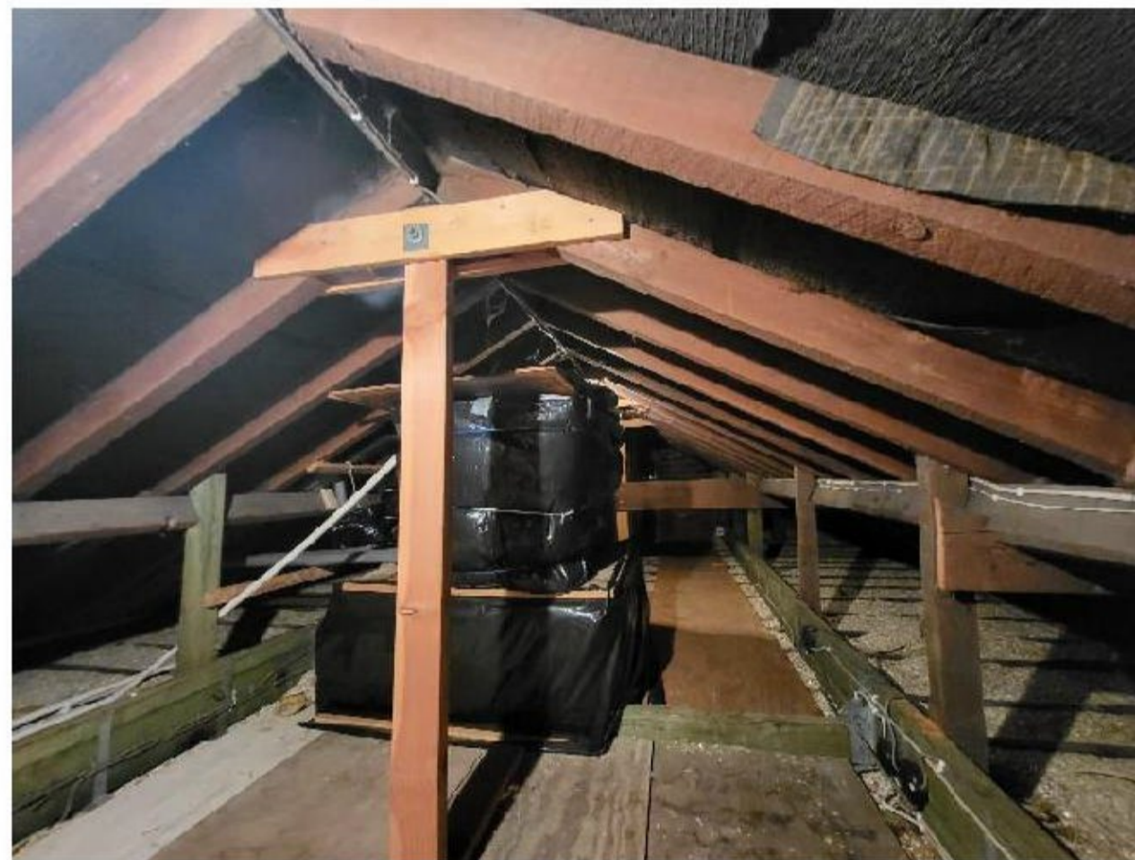
Figure 10. View of the loft
