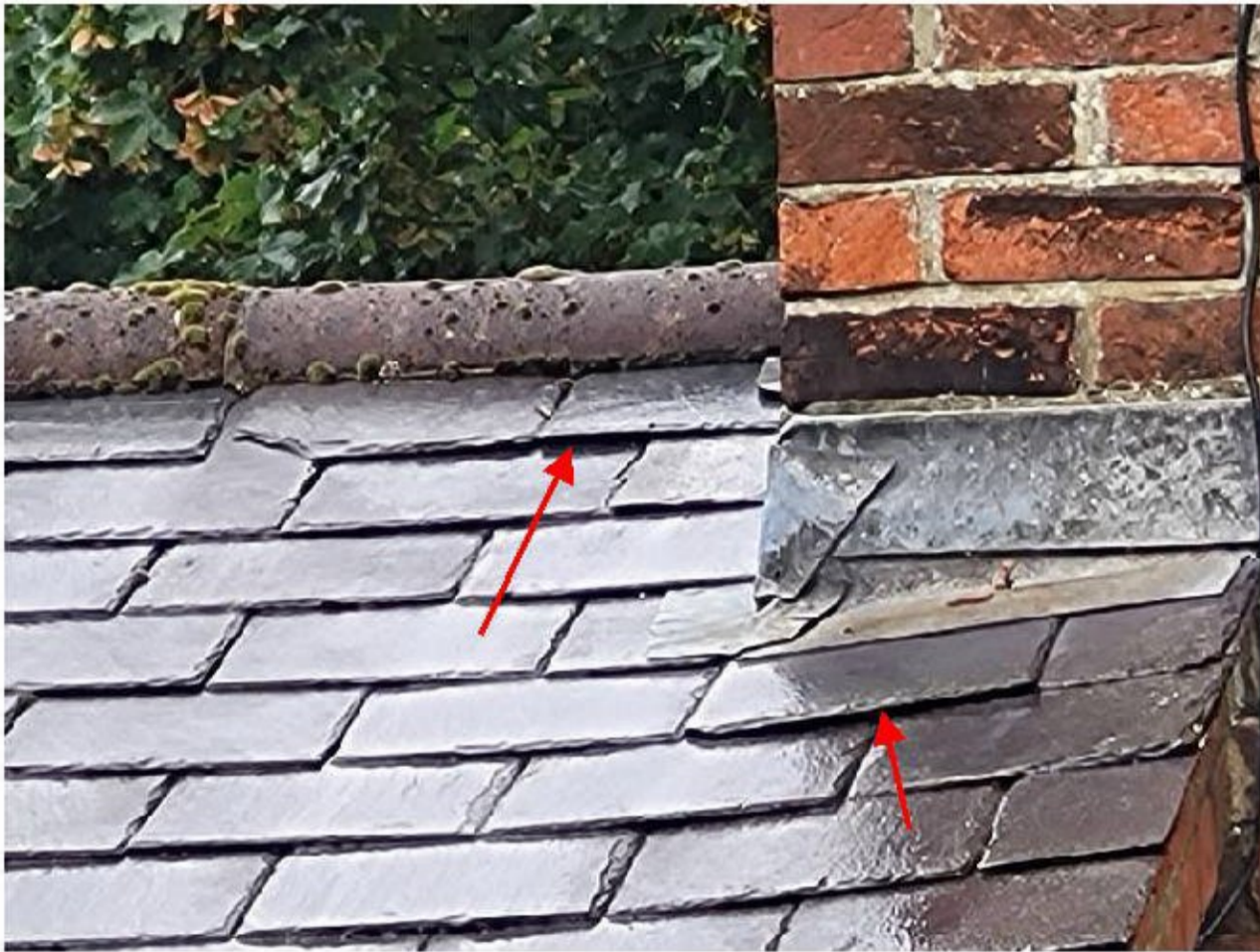
Figure 6. Example of slightly lifted roof slates
