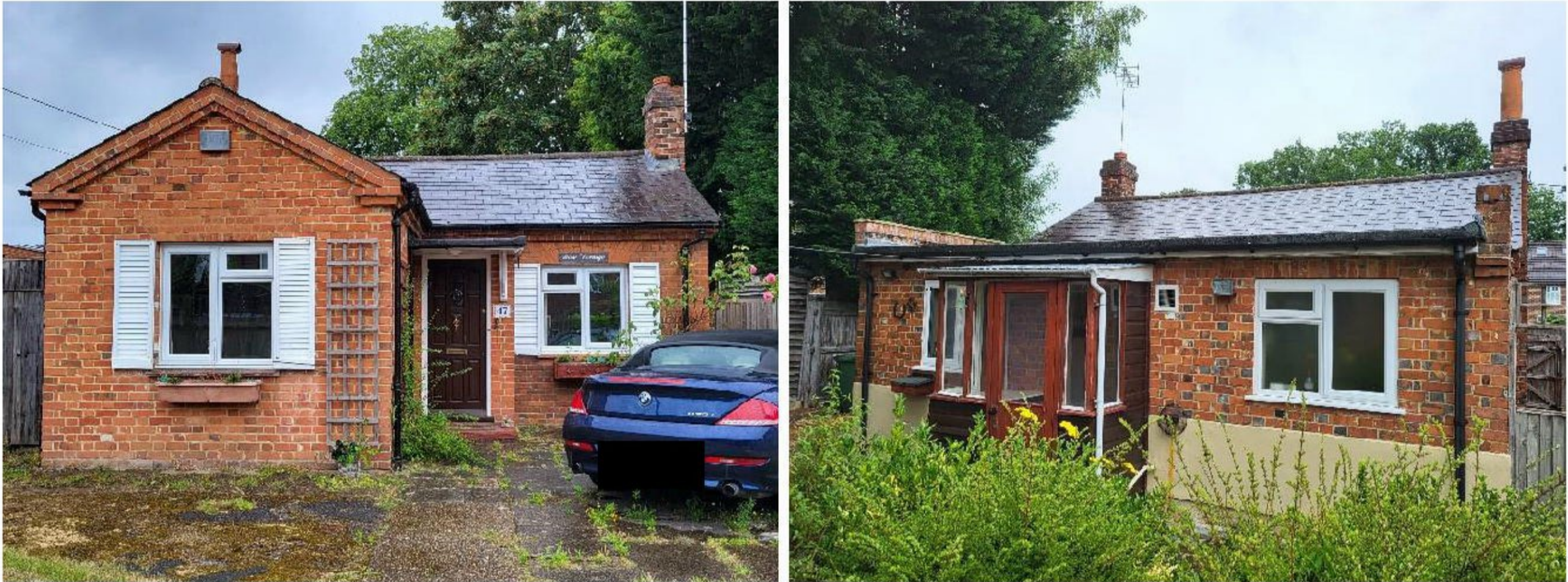
Figure 2. View of the front and rear elevations of the dwelling
