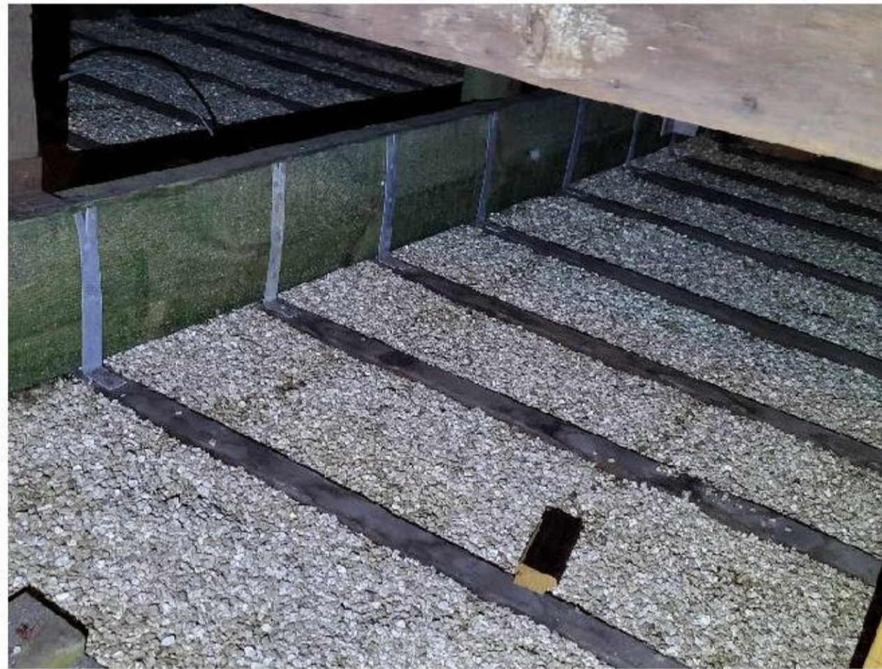
Figure 13. View of the loose fill insulation
