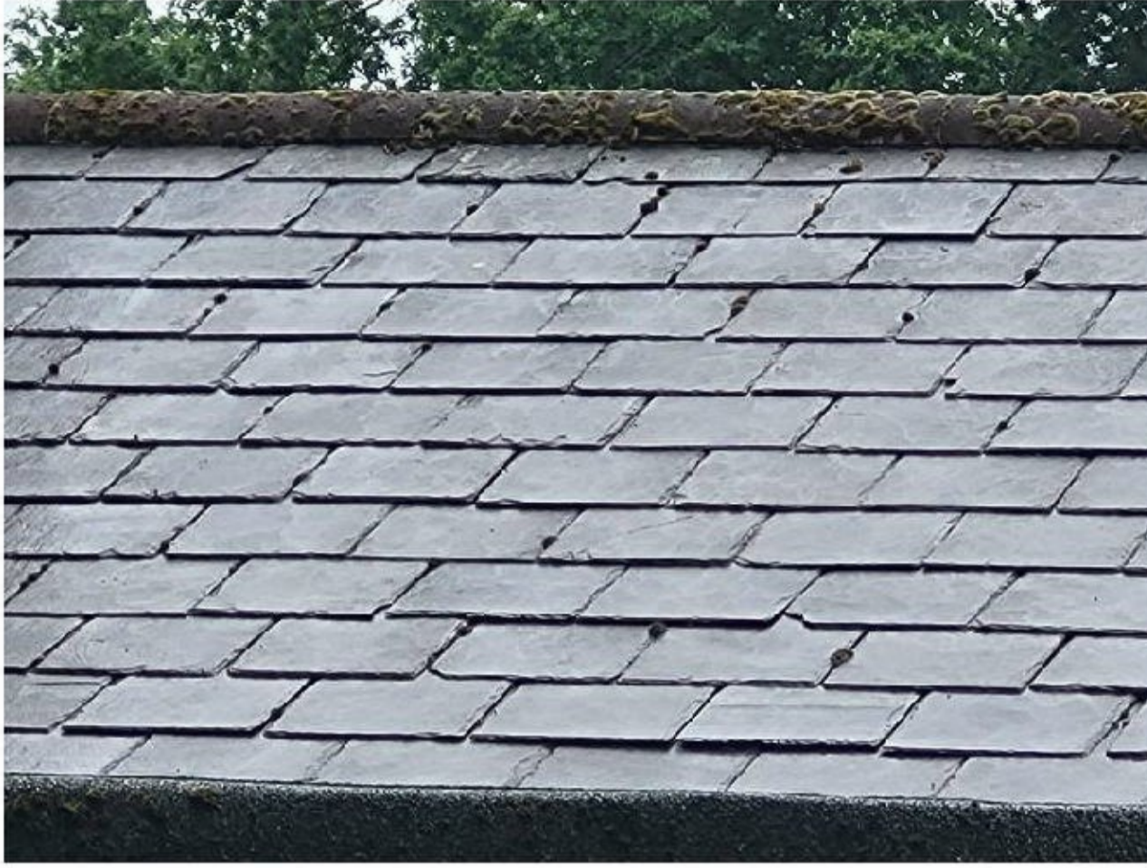
Figure 4. Example of tightly fitted roof slates
