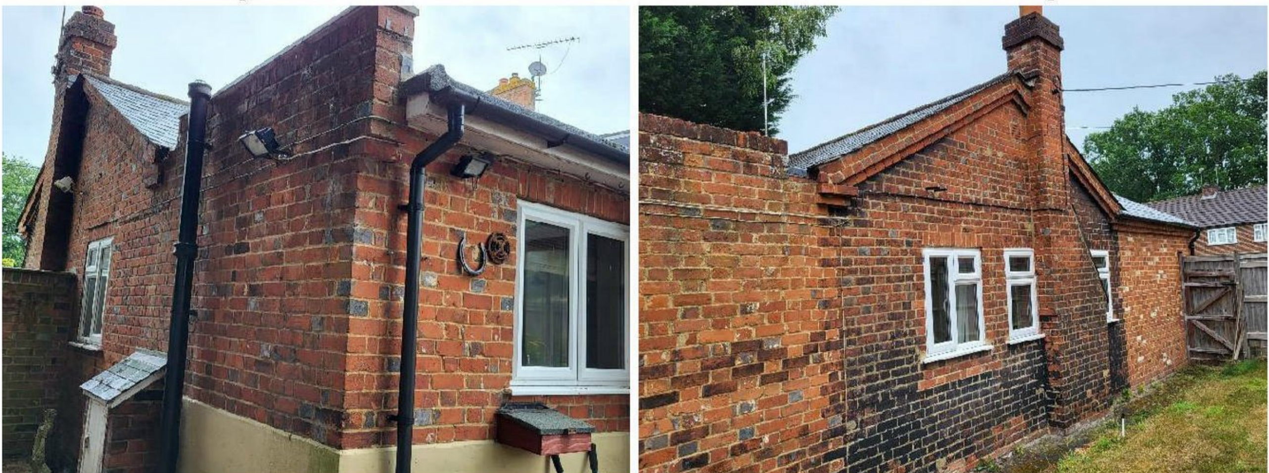
Figure 3. View of the side elevations
