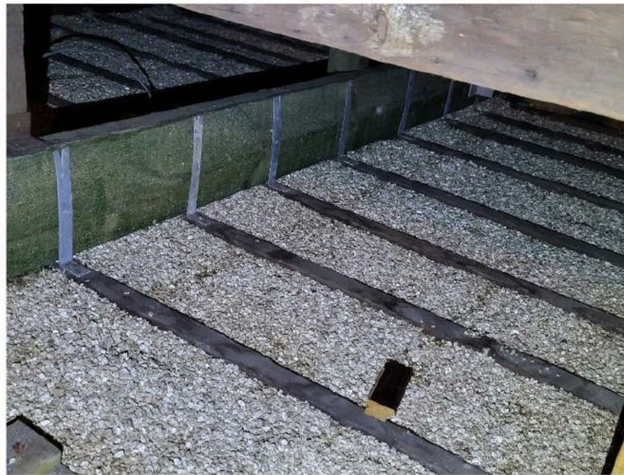
Figure 13. View of the loose fill insulation
