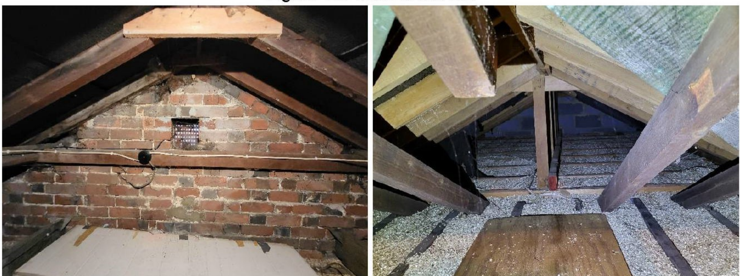
Figure 11. View of the brick and breezeblock gable-ends
