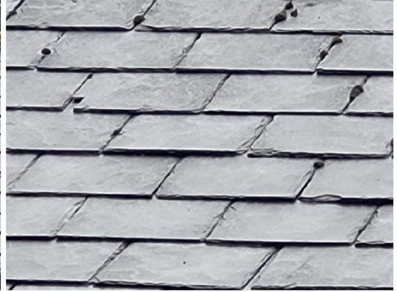
Figure 4. Example of tightly fitted roof slates
