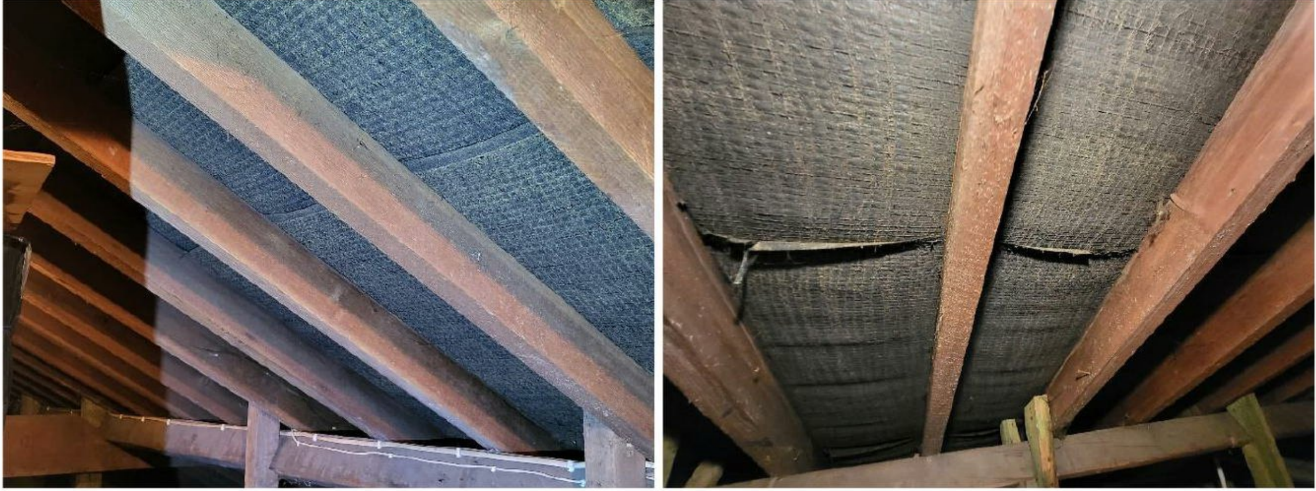
Figure 12. View of the roofing felt between rafters and slates
