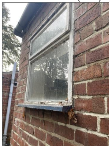
Window 2 – kitchen rear (east) elevation
