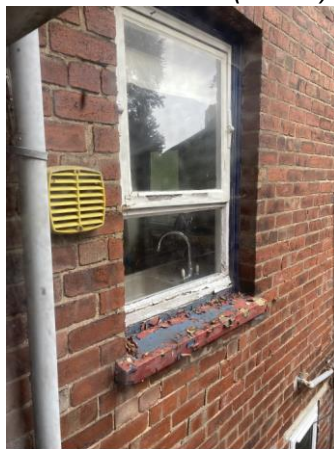
Window 1 – kitchen side (south) elevation
