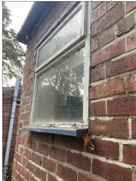
Window 2 – kitchen rear (east) elevation
