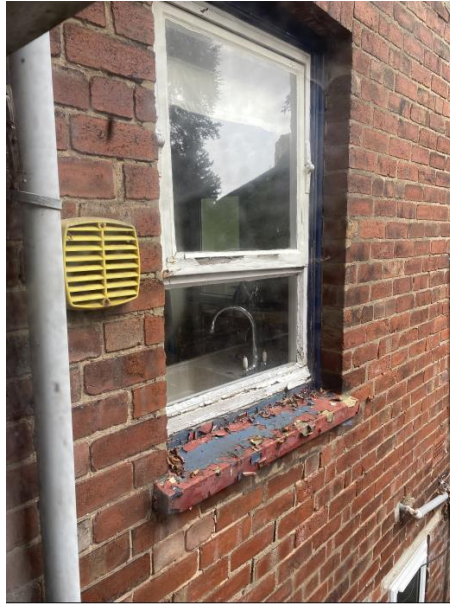
Window 1 – kitchen side (south) elevation
