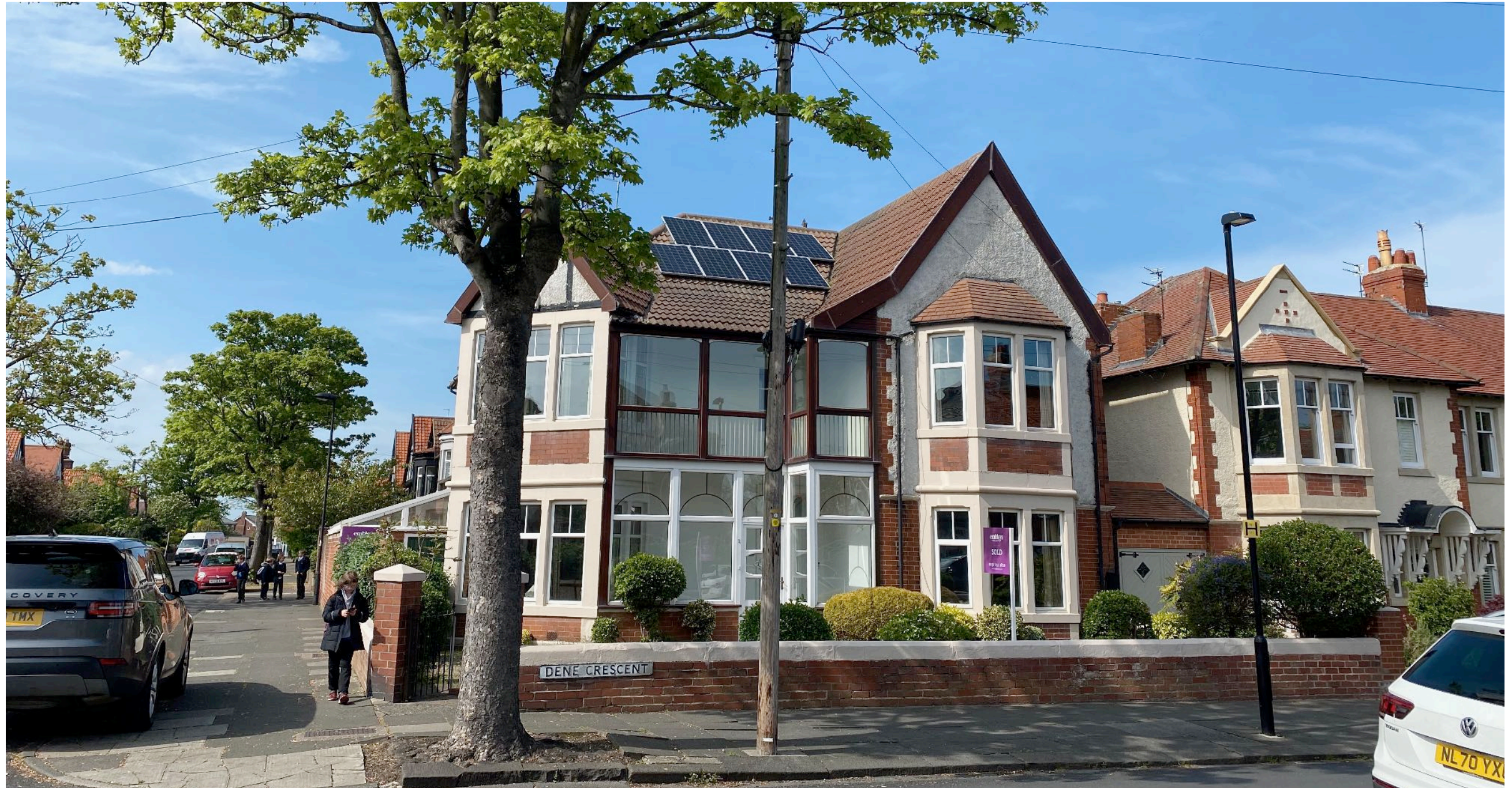
Heritage, Design and Access Statement : 2 Dene Crescent, Whitley Bay. NE26 3AL
