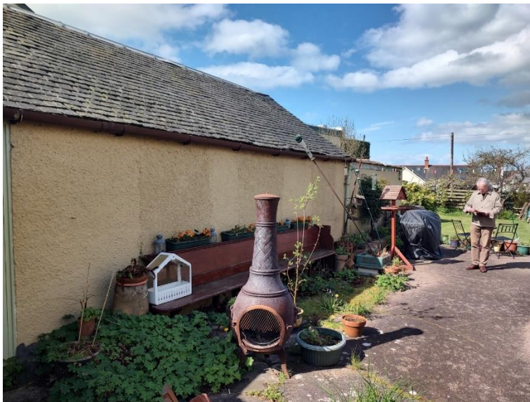
Rear of retail unit and garden store; soft landscaping beyond.
