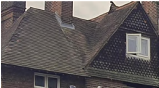
Dentils to eaves and herringbone tiles on gable
