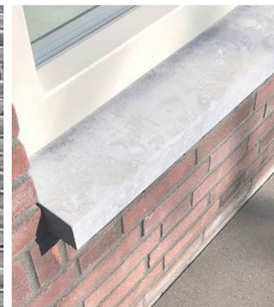
3. Light coloured stone cill
