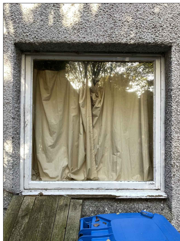
WINDOW TAG 3 - EXTERNAL VIEW
