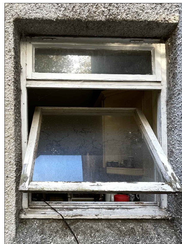
WINDOW TAG 4 - EXTERNAL VIEW
