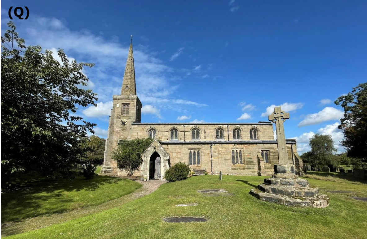
Figure 25: Well outside the application site, the frontage (Southeast Elevation) of the Nearby Grade I listed St. Michael's Church. Some aspects of the Church are as old as C12 late Norman period (1066-1154); however, the Church is C14 in the main, with some C15 aspects. The Spire, which is the only feature seen from the application site, is a C14 recessed spire.
