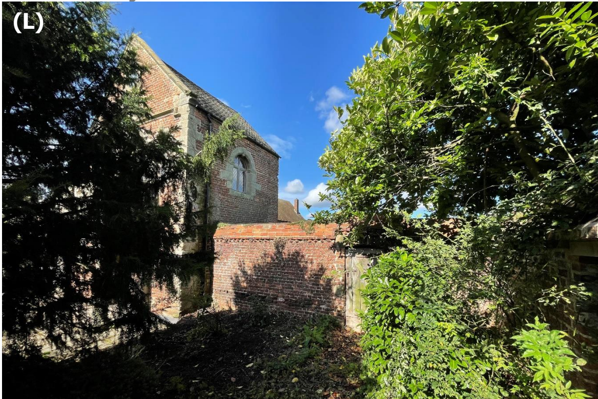
Figure 20: From 'Side Garden' looking North. St. Michael's Church to the right-hand boundary. Looking at the Side Elevation of the Gable / Loggia from C16. This has exterior windows suggesting that the original Hall would have begun beyond the rear of this surviving structure and the Garden Wall in the foreground was not a former wall.
