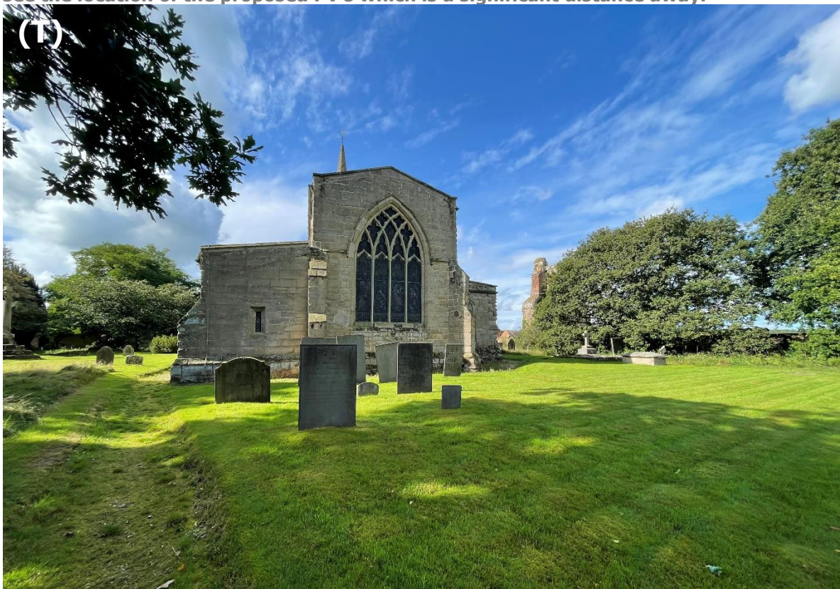
Figure 28: The East facing Elevation at St. Michael's. Here we see the early C14 chancel with pointed east window of four trefoil-headed lights and cusped intersecting tracery.
