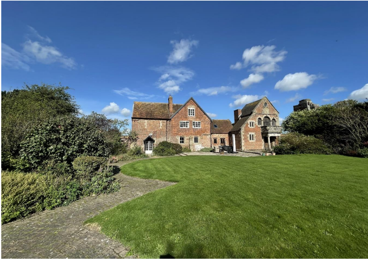
Figure 33: Strategic Option 2 – Central in the 'rear area' of the 'side garden' alongside Hamstall Hall to the South.
