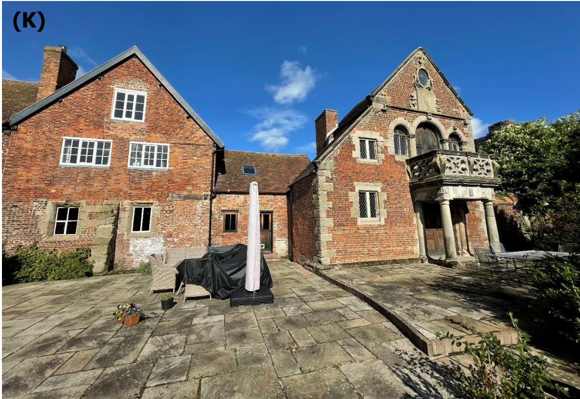
Figure 19: The Side Elevation of Hamstall Hall; as a Grade II* listed building this is of "more than special interest". Across the Elevation greater significance can be attributed to the right-hand Gable and Porch which are heavily embellished and provide an insight into what the C16 Hamstall Hall would have been like architecturally. Aspects to the left-hand side are thought to date from a substantial rebuilding around 1821.
