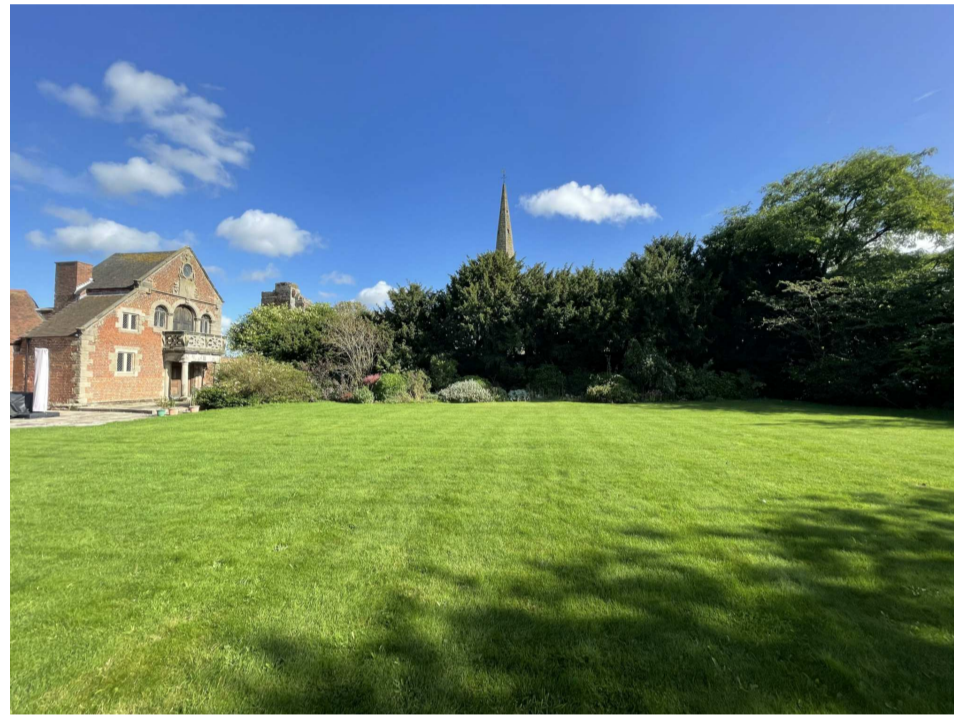
Photo 9 From the back part of the 'side garden'. In this photo we can see the original C16 bay of Hamstall Hall and the C14 Church Spire in the background. We can also see the dense vegetation which separates St. Michael's Church from the application site.
