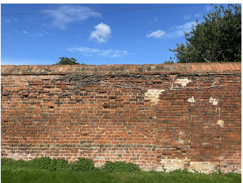
Photo 8 The 'Garden Walls' as described in 'Photo 7'. These are Grade II Listed and have evidential, historic and aesthetic significance. Condition is fair given its age, although some aspects are poor and repairs have been carried out in multiple phases.
