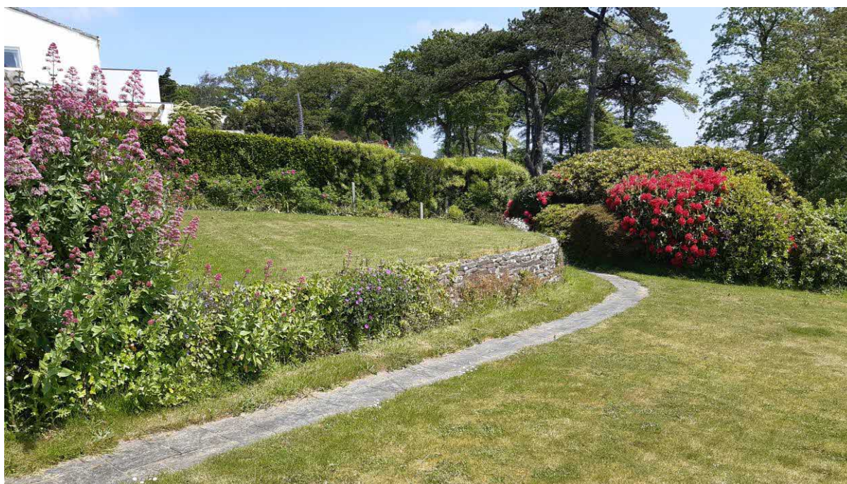
Figure 5: View looking north of the retaining garden walls with vegetation cover
