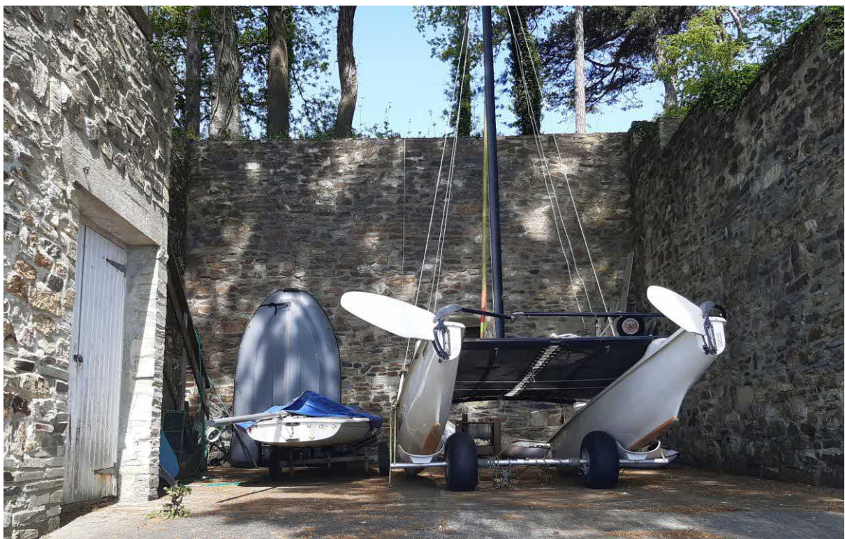
Figure 4: Retaining walls around boatyard area with adjacent storage building
