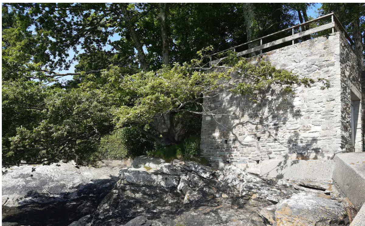
Figure 2: View looking southwest of the storage building with adjacent foreshore.
