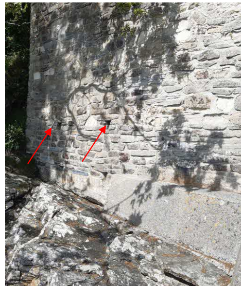
Figure 10. Pipe openings in store building
