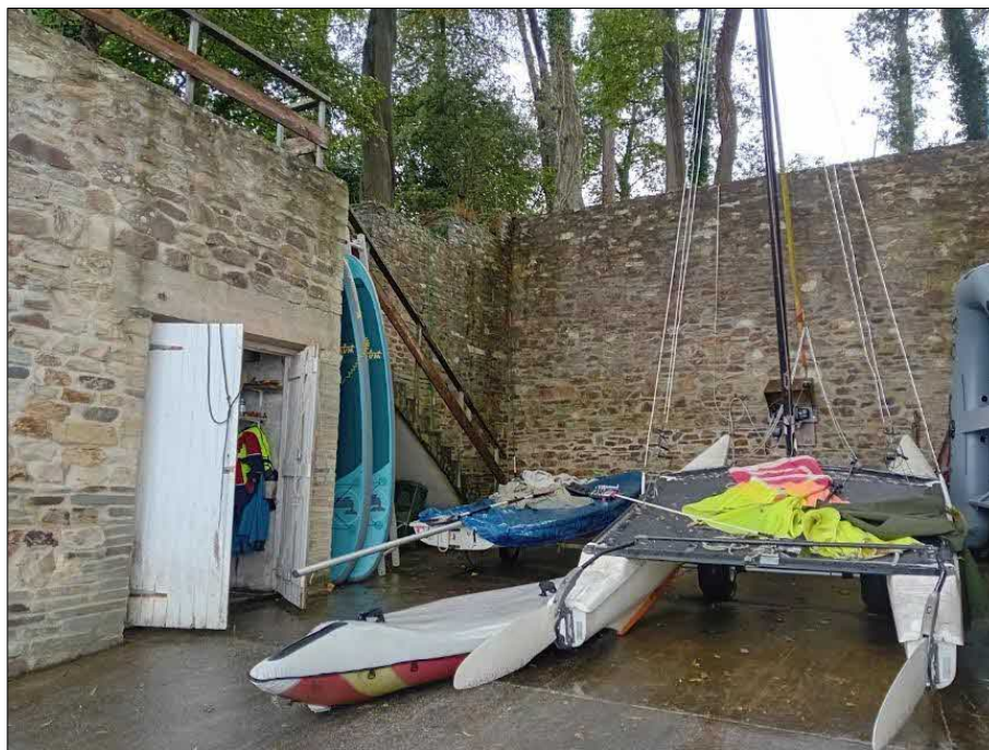
Figure 04: The existing boat storage area, from the beach looking west.
