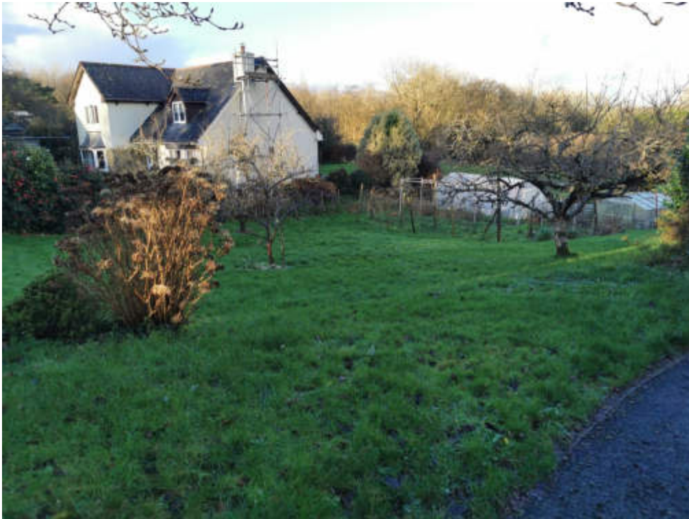
Plate 1: Overview of development area looking northwest.
