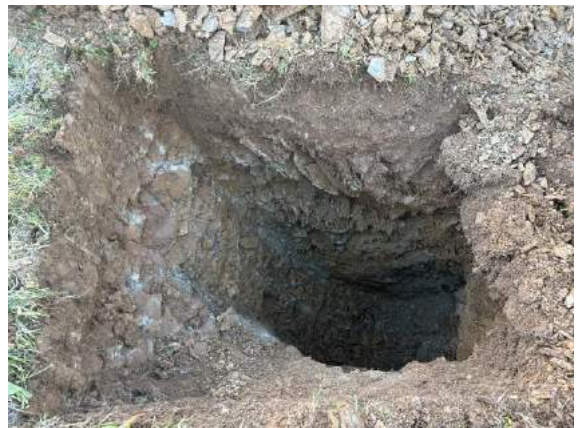
Photo 16: Completed TSAH from Face C looking 240 SW
