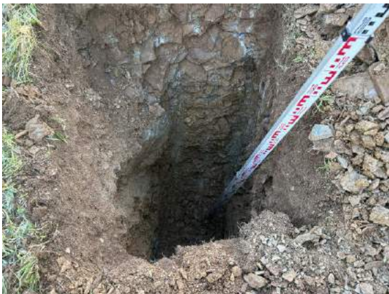
Photo 15: Completed TSAH from Face A looking 150 SE
