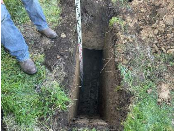
Photo 1: Completed TP01 from Face B looking 010 N
