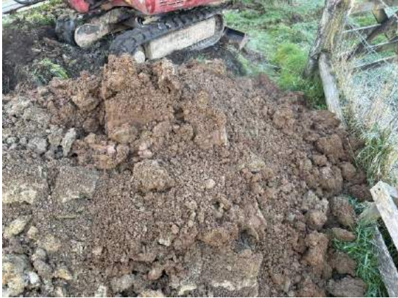
Photo 7: Spoil of TP01 (0.90 – 1.60m) looking 010 N
