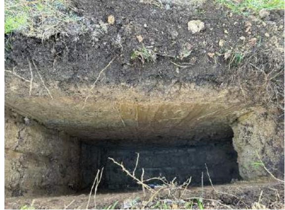
Photo 2: Completed TP01 from Face A looking 280 W
