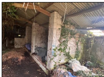
Internal structure of Barn 2
