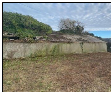
Western elevation of Barn 2
