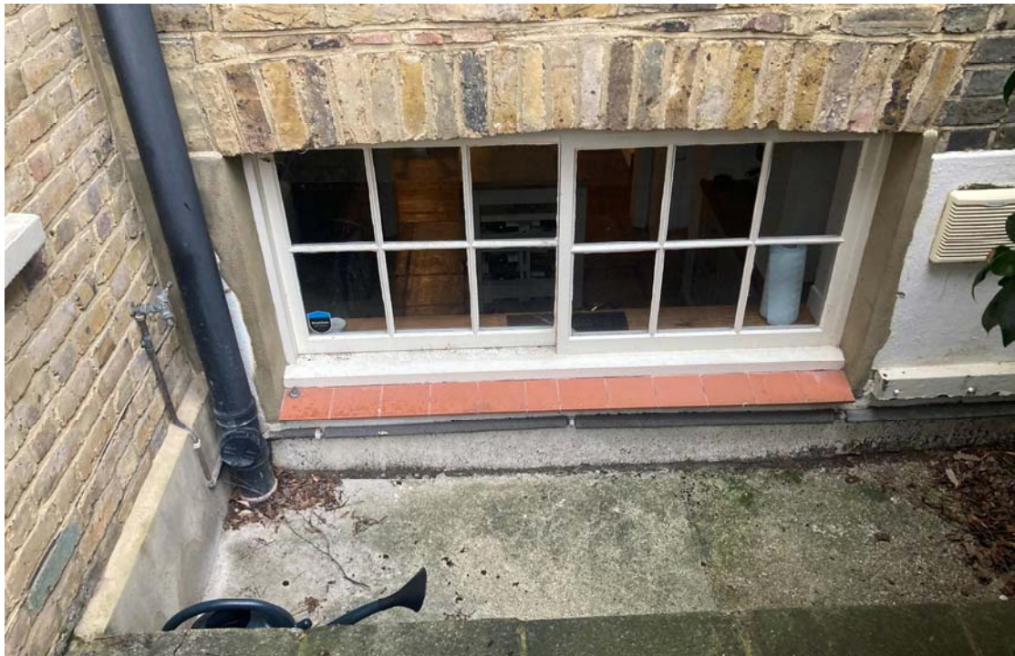
Photo 3: Rear basement window to be demolished
