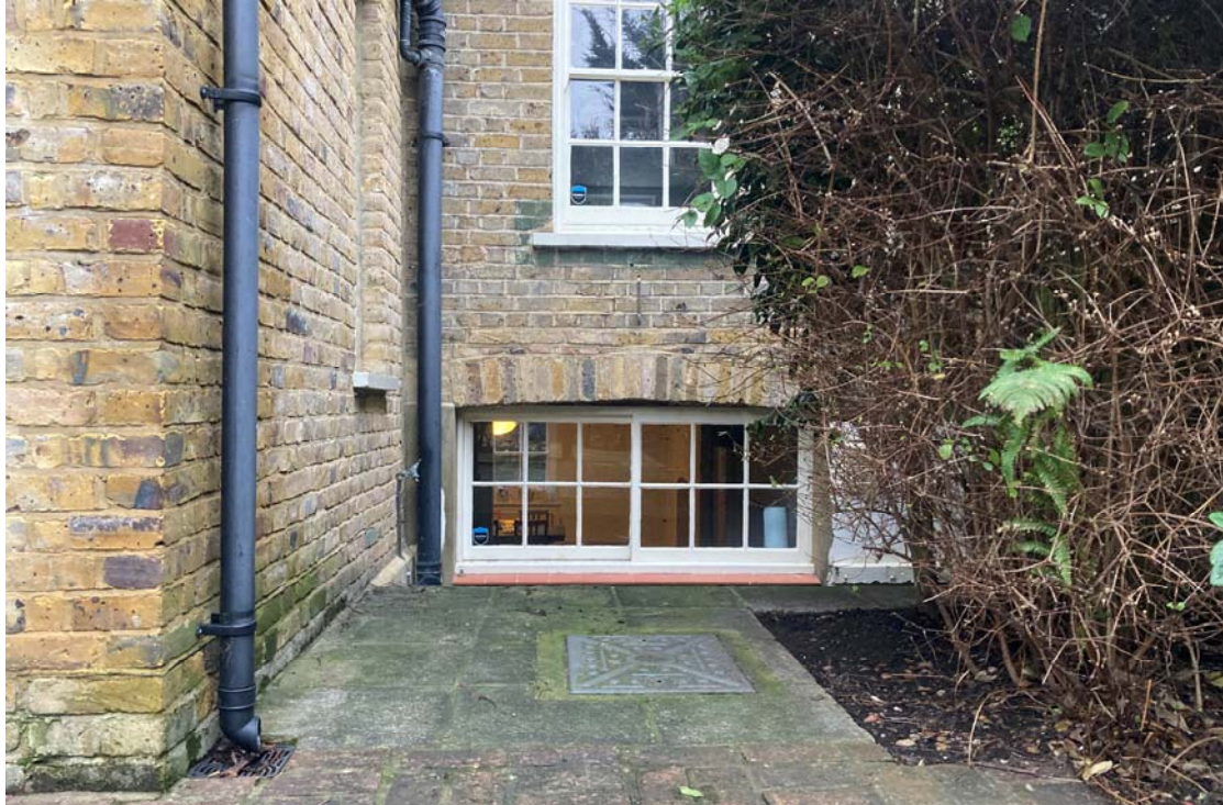
Photo 2: Rear basement window to be demolished
