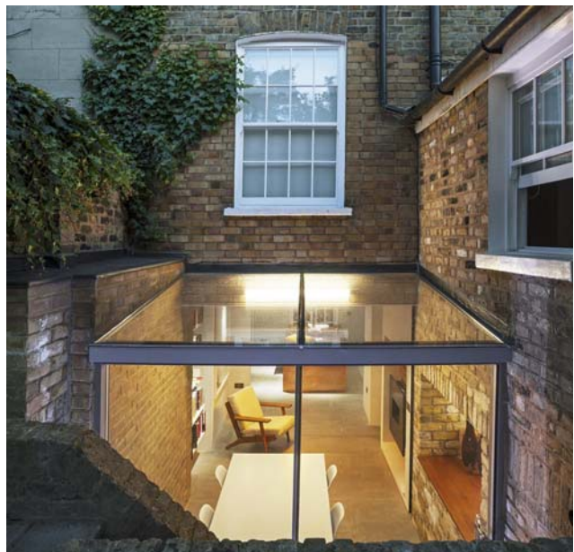
Photo 6: Sunken glass box extension to heritage-listed London house by Space Group Architects
