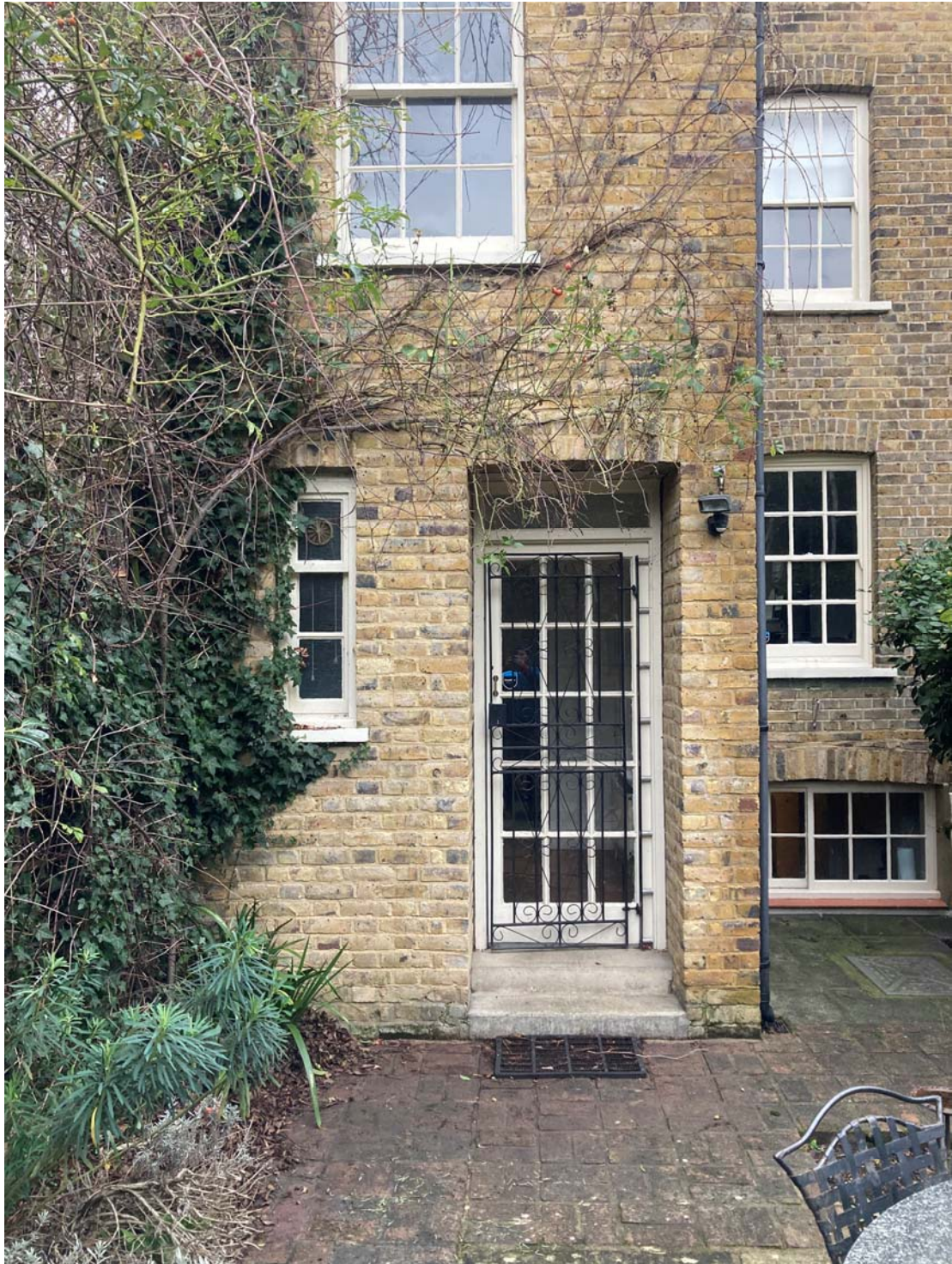
Photo 12: View of rear elevation
