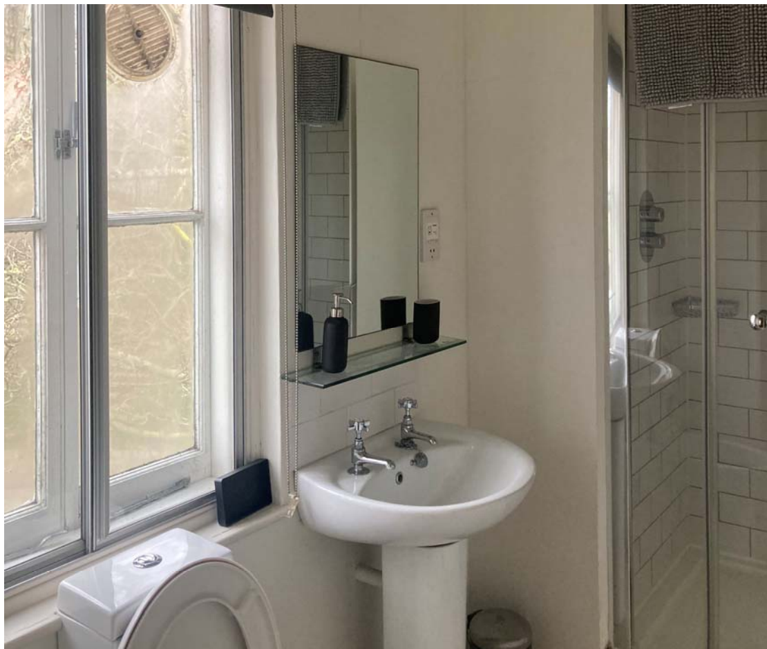
Photo 14: Second floor bathroom to be demolished
