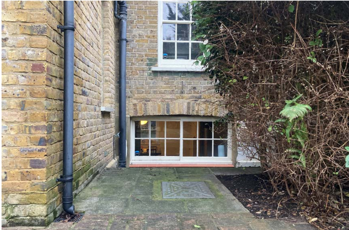
Photo 6: Rear basement window to be demolished
