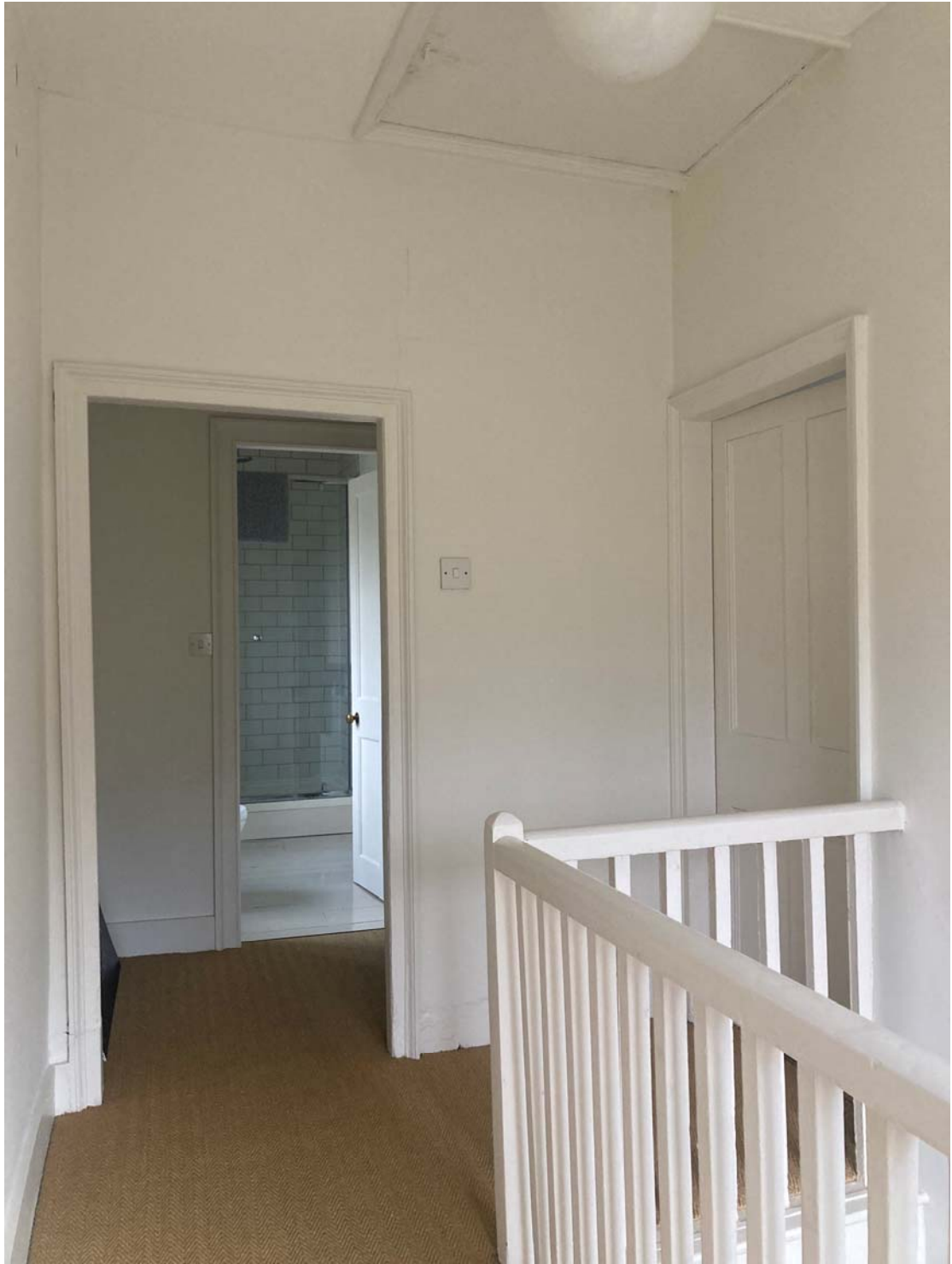
Photo 16: Second floor landing, view to bathroom to be demolished
