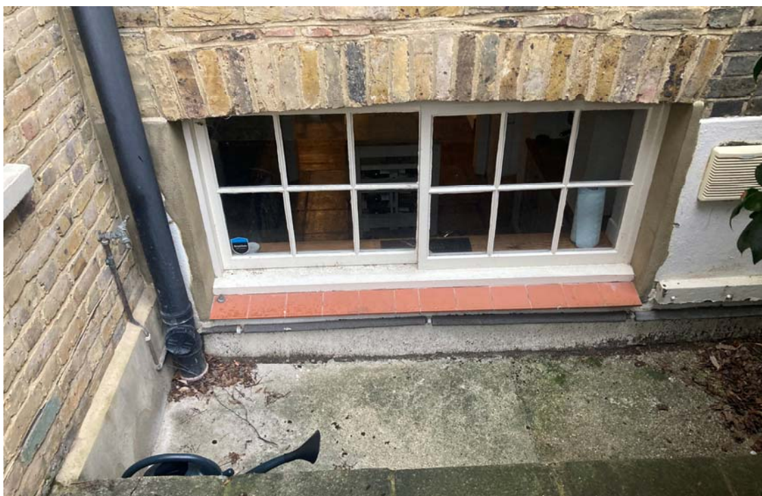
Photo 7: Rear basement window to be demolished
