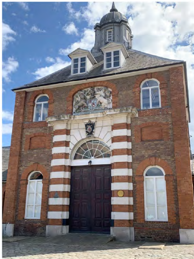
Plate 1: Royal Woolwich Arsenal viewed from the River (north)
