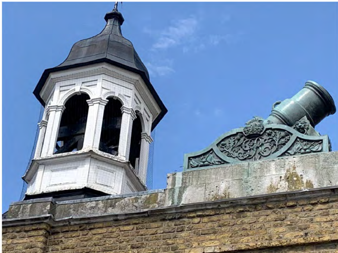
Plate 10: Detail to Main Entrance Gates
