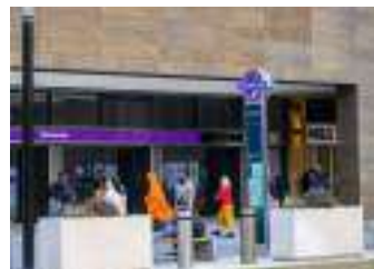
2. Woolwich Arsenal Elizabeth Line Station
