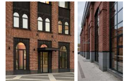
Precedent image. Contrasting brick and black fenestration
