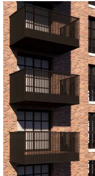
① Metal balcony fascia and railing balustrade
