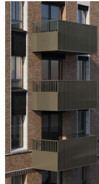
③ Metal balcony fascia, front railing balustrade and combined solid side metal balustrade with railing
