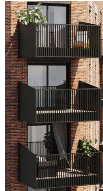
② Metal balcony fascia, front railing balustrade and side metal panels
