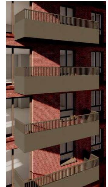
④ Metal balcony fascia and combined solid metal balustrade with railing
