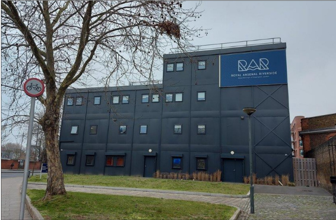
PHOTOGRAPH 1: Building B1 southern elevation
