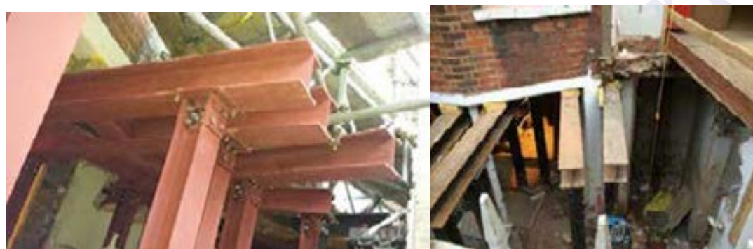
Figure 1 Example of needling to existing wall
