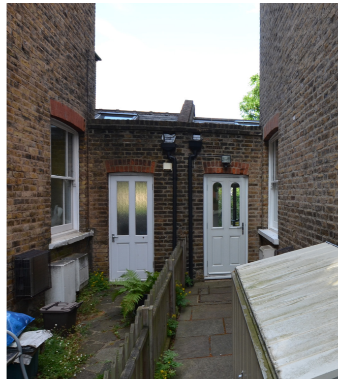
Alleyway to side entrance
