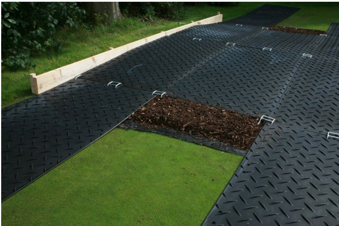
Figure 4. Example of propriety inter-linked ground protection boards placed on top of a compression-resistant layer (e.g. 150 mm depth of woodchip), laid onto a geotextile membrane, suitable for pedestrian-operated plant up to a gross weight of 2 t
