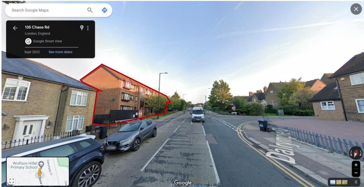
Figure 19: On Chase Road leading up to the site, Grovebury Court on the left. As can be seen, the road surface and footways are uneven due to roadworks.
