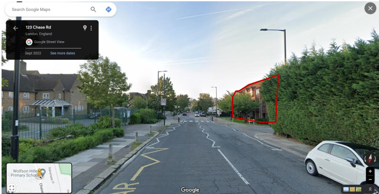
Figure 20: On Chase Road with the site on the right.
