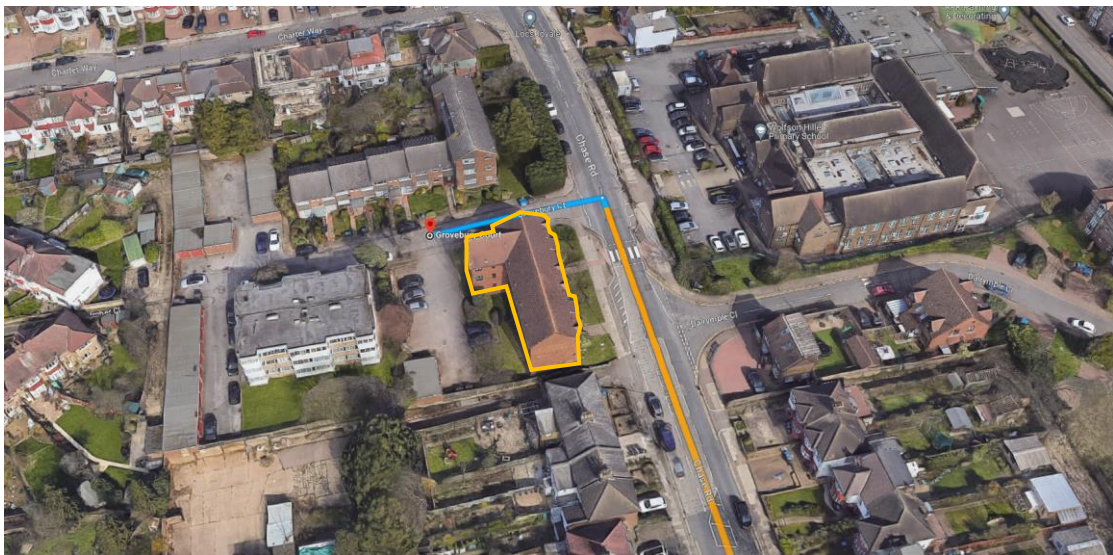
Figure 3: Ariel view of the proposed site at Building A, 33-47 Grovebury Court, London, N14 4JR. It is proposed to have 1 additional storey on the existing block of flats. As can be seen, Wolfson Hillel Primary School is located adjacent to the development.
