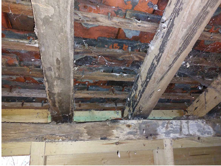
Image 07 – View of roof tiles from interior of lean-to structure.
