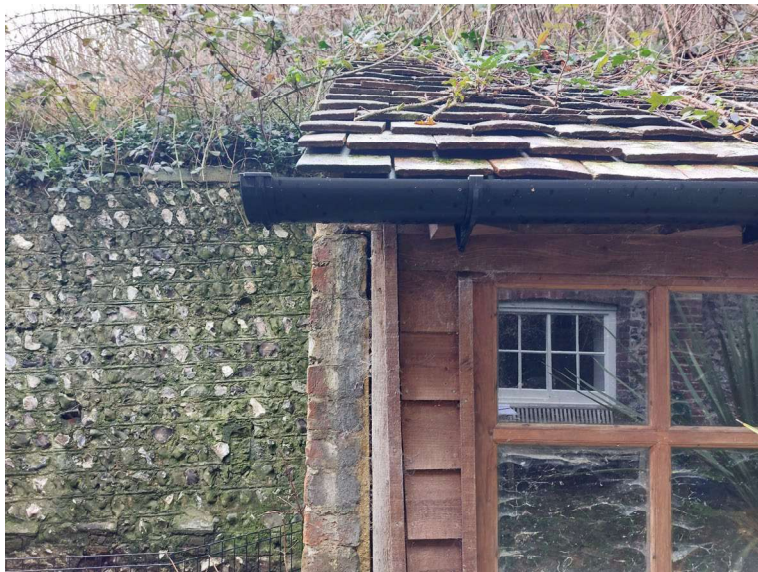
Image 04 – View of PRF between brick side wall and front timber structure.
