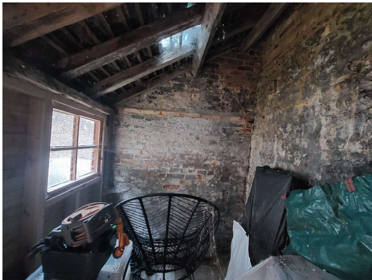
Image 06 – View of interior of lean-to structure.
