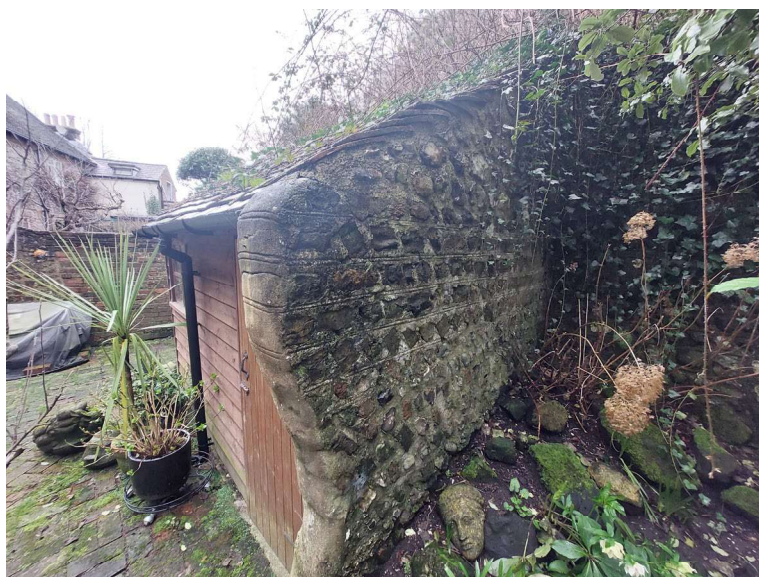
Image 02 – View of historic flint wall.
