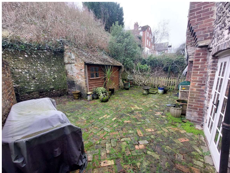
Image 01 – View of entire site north to south, with lean-to scheduled for demolition in centre of image, residential dwelling to the right of image.
