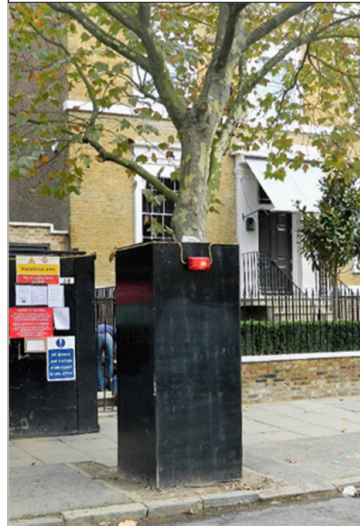
b) Stabilizer strut mounted on block tray
