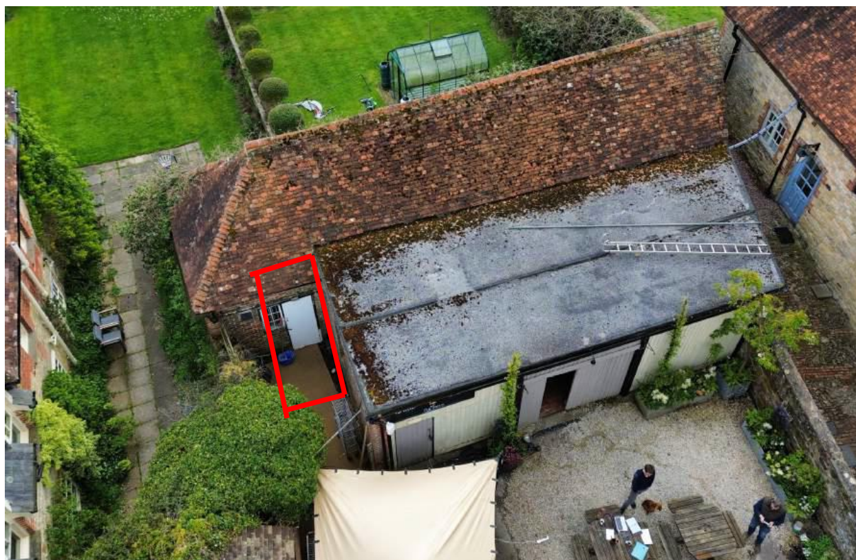
Photograph No 1- the site for the proposed zinc roof outlined in red. The grey roofed building has permission to be demolished under SDNP/23/0208/Ful & SDNP/23/02029/LIS.
