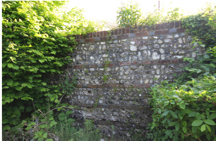
Boundary wall from Tyne House side
