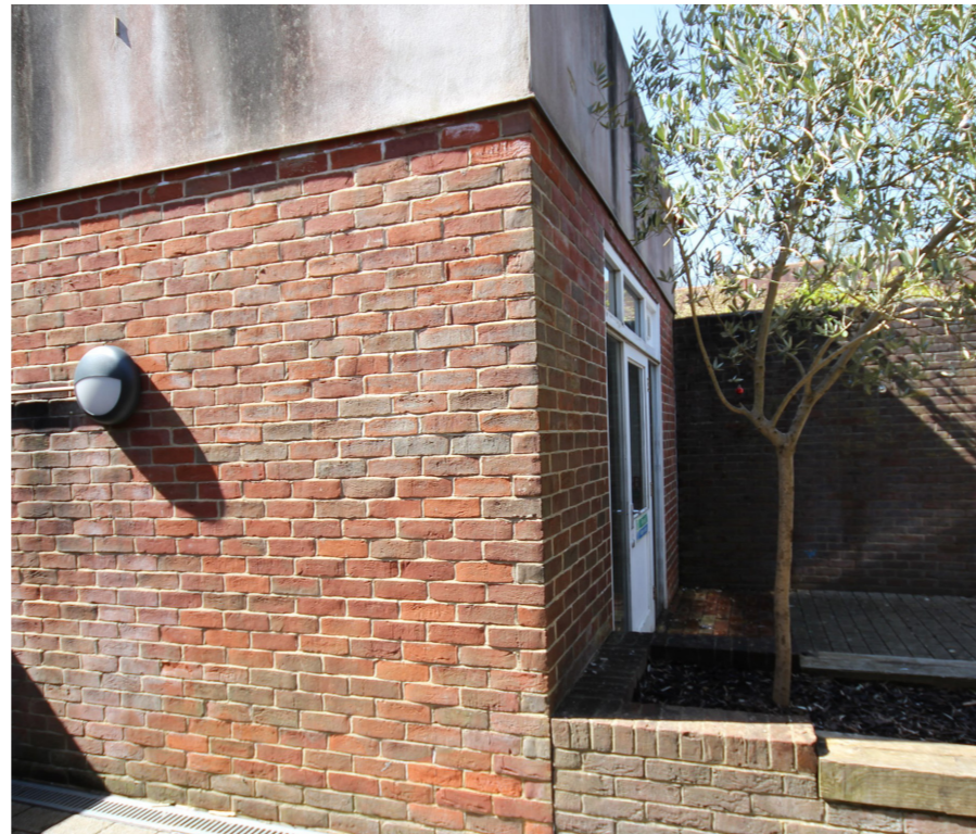
Existing extension to St Clair House
