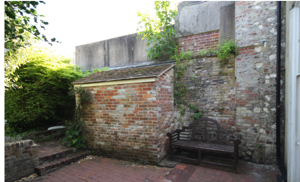
Boundary wall from Tyne House side
