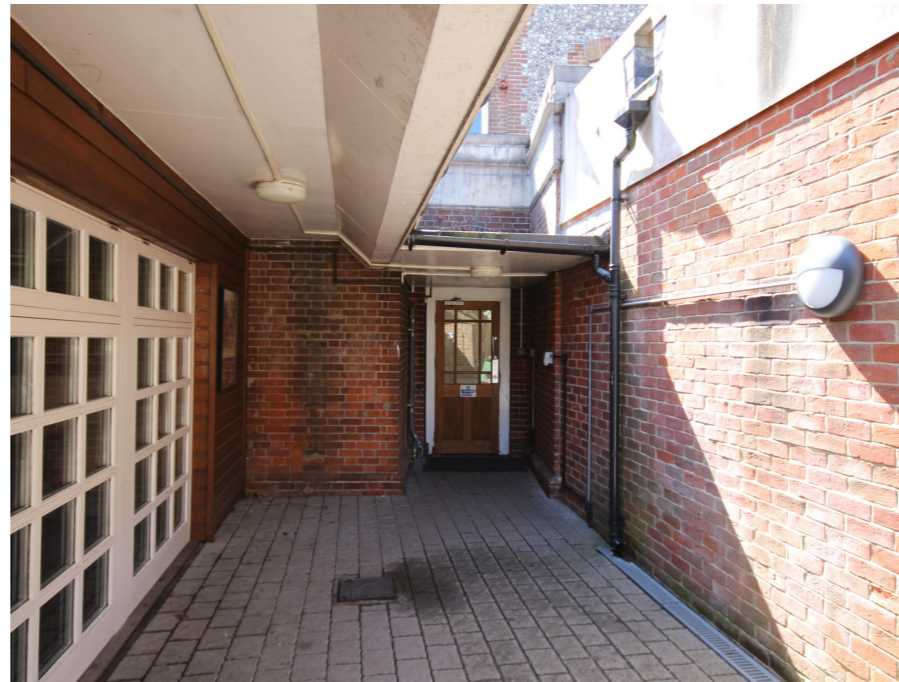
Existing access between St Clair and The Malling
