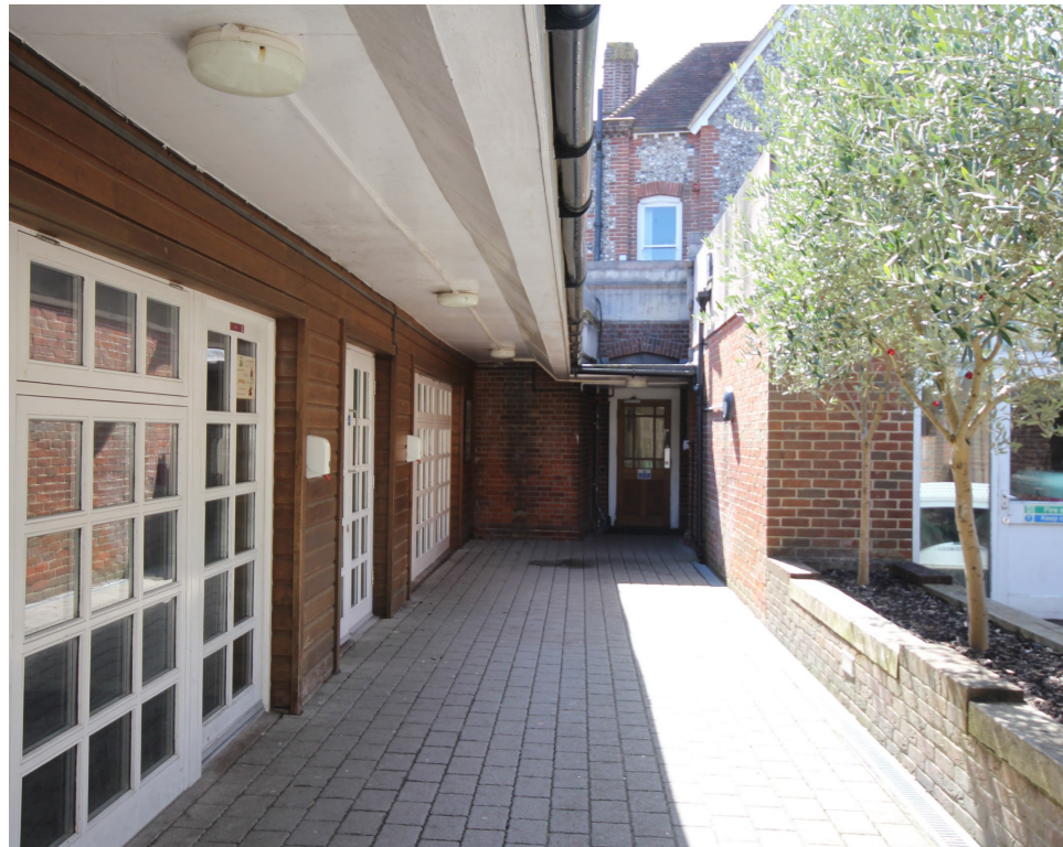
Existing access between St Clair and The Malling
