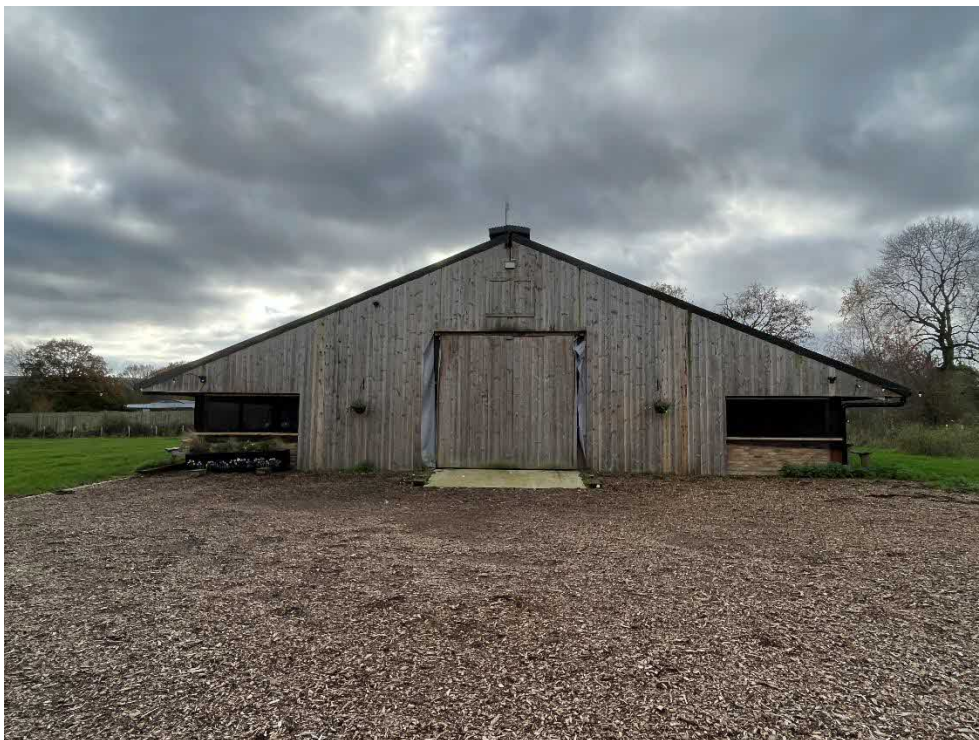
Photo Above: The Application Barn
