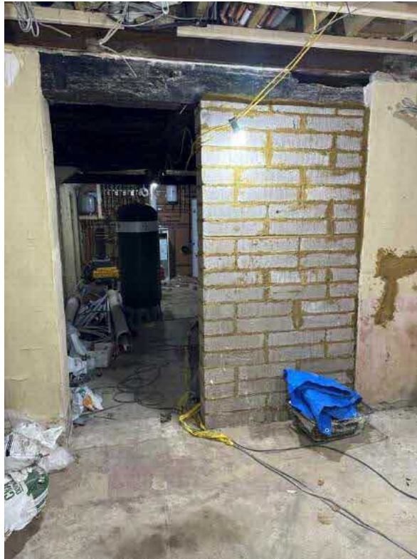
Plate 16. Probable re-used beam between the rear wall of the house and the outbuilding.
