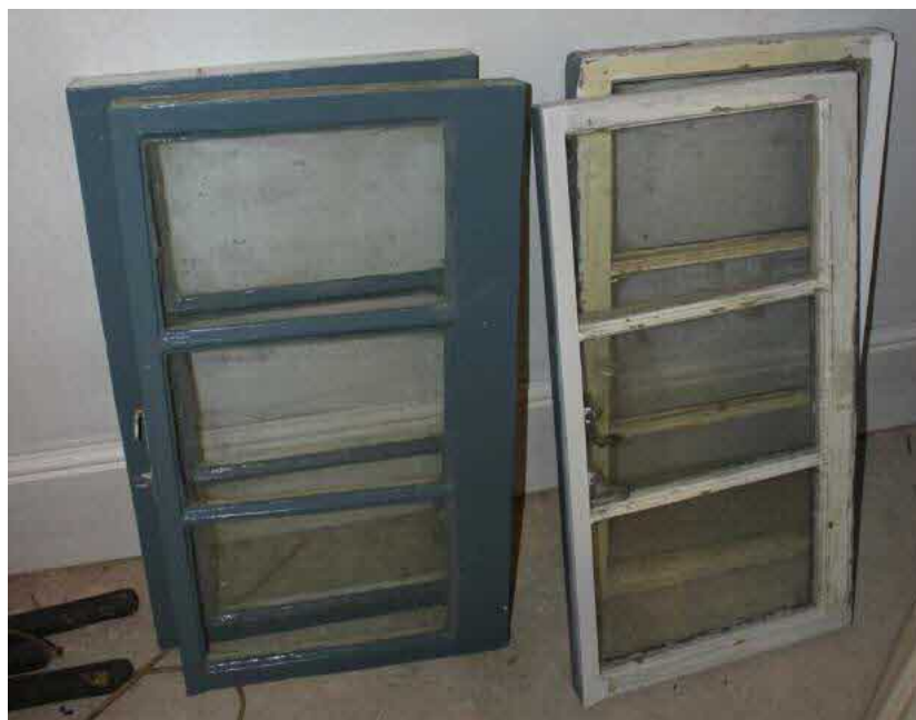
Plate 21. Repaired sashes from the ground floor window.
