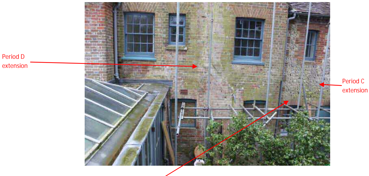
Plate 18. Single segmental brick lintels in the Period C extension.
