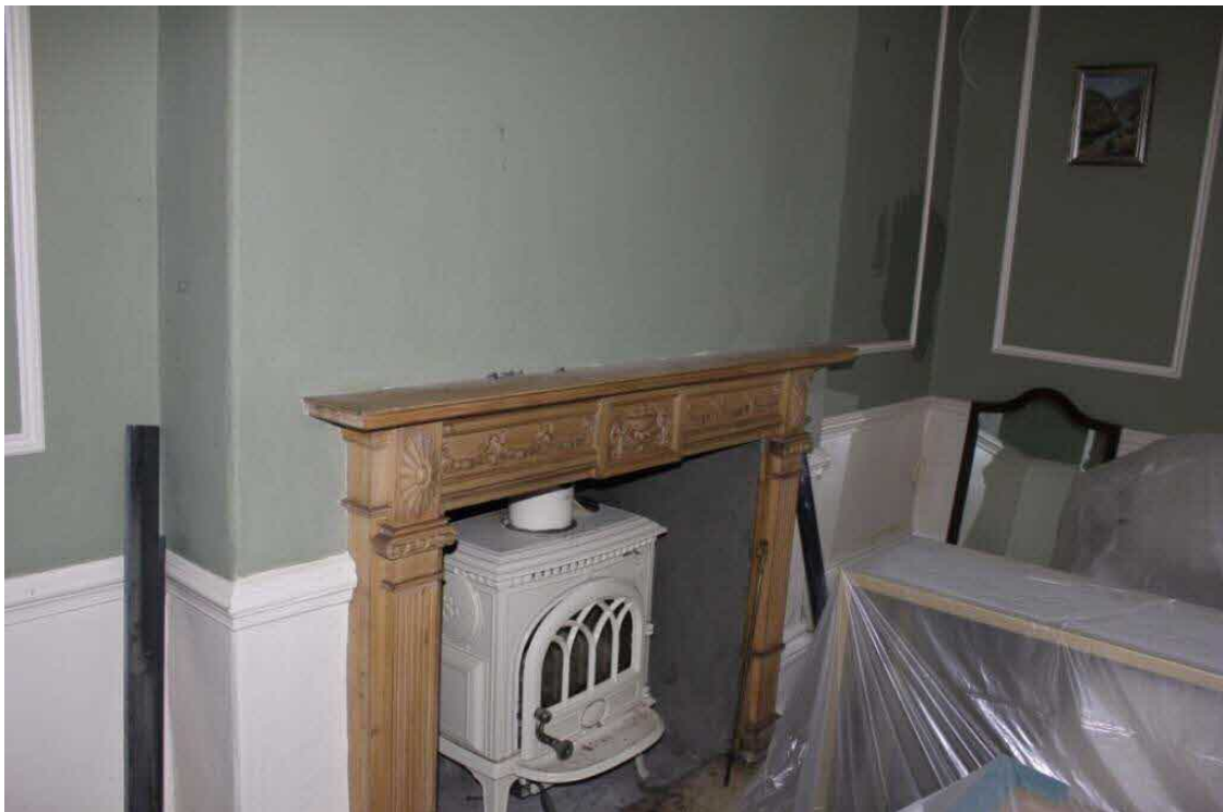
Plate 30. Fireplace surround in the high status drawing room.
