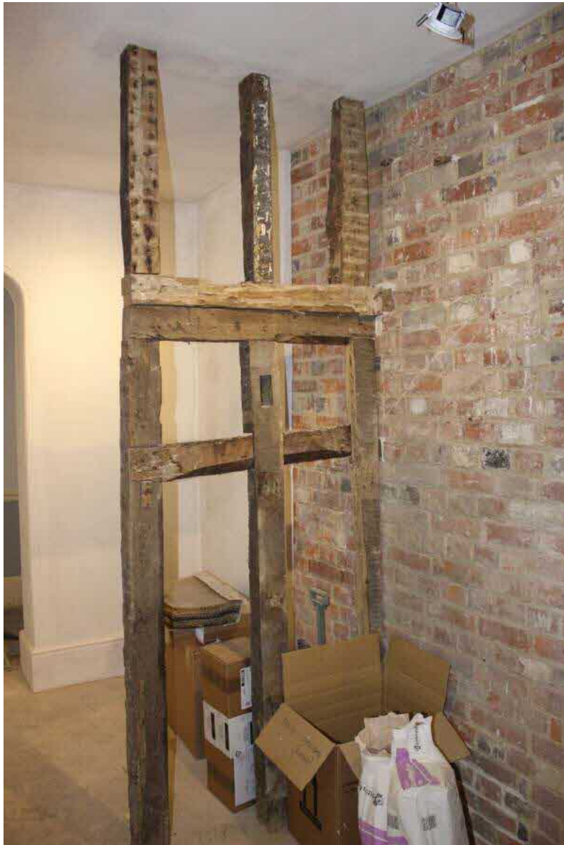
Plate 15. Makeshift stud wall using recycled timbers at ground floor.
