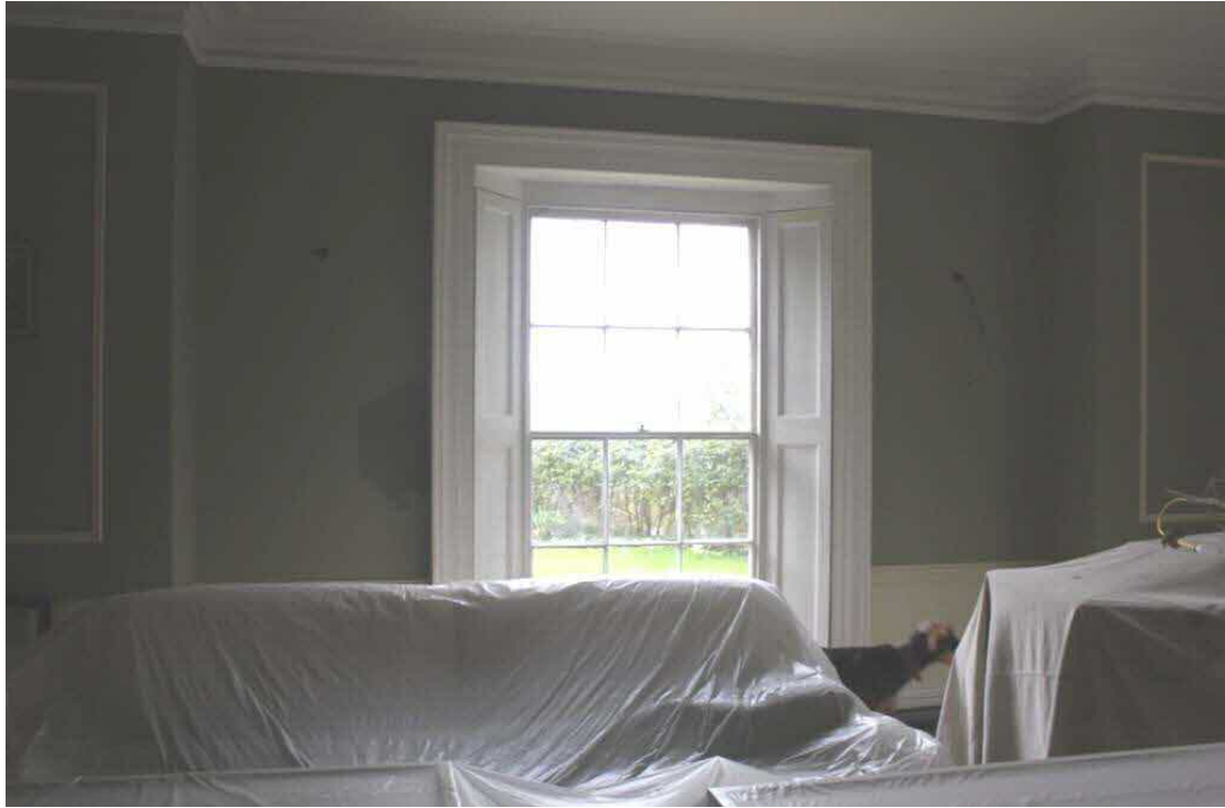
Plate 29. Eastern window with shutters.
