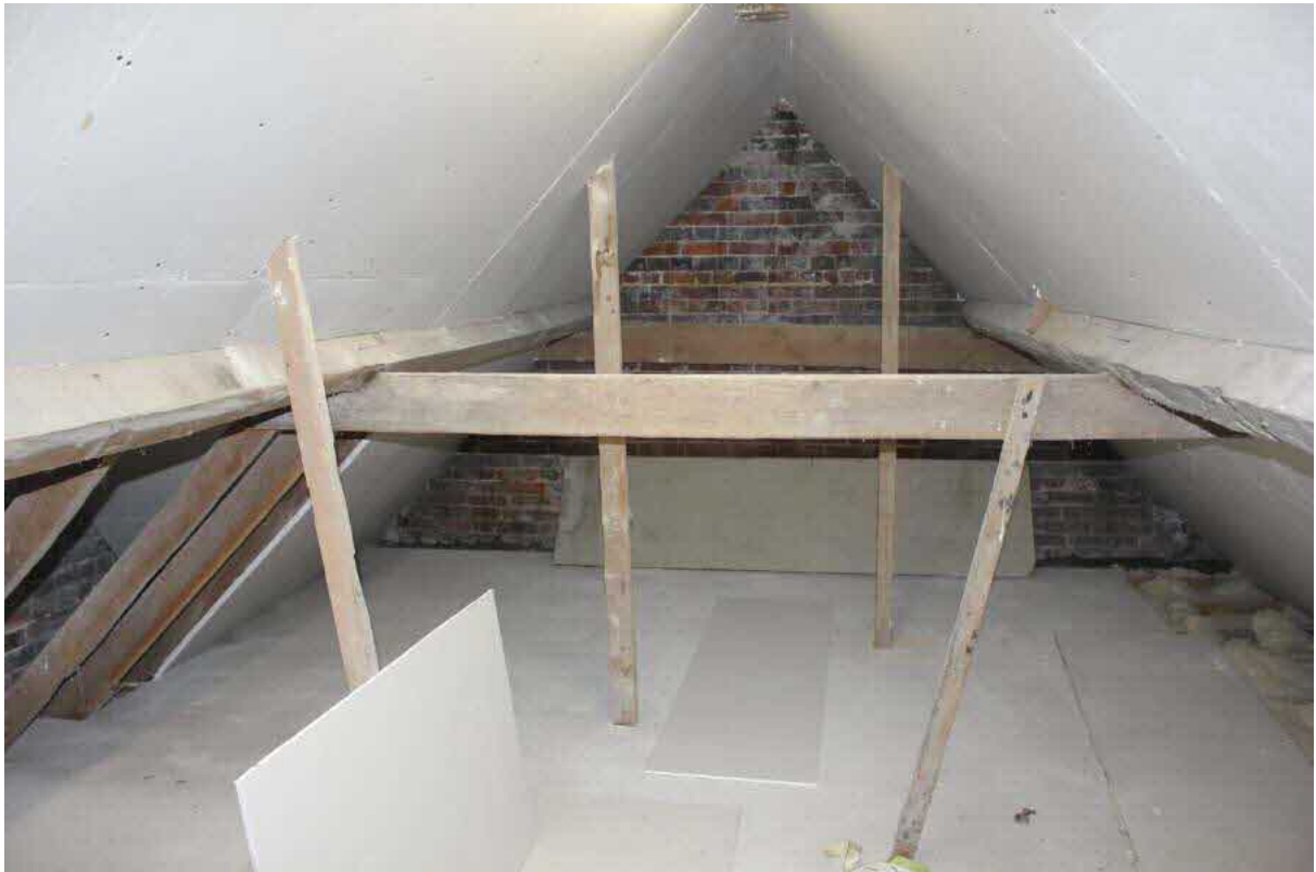
Plate 33. The roof of the high status wing looking south.
