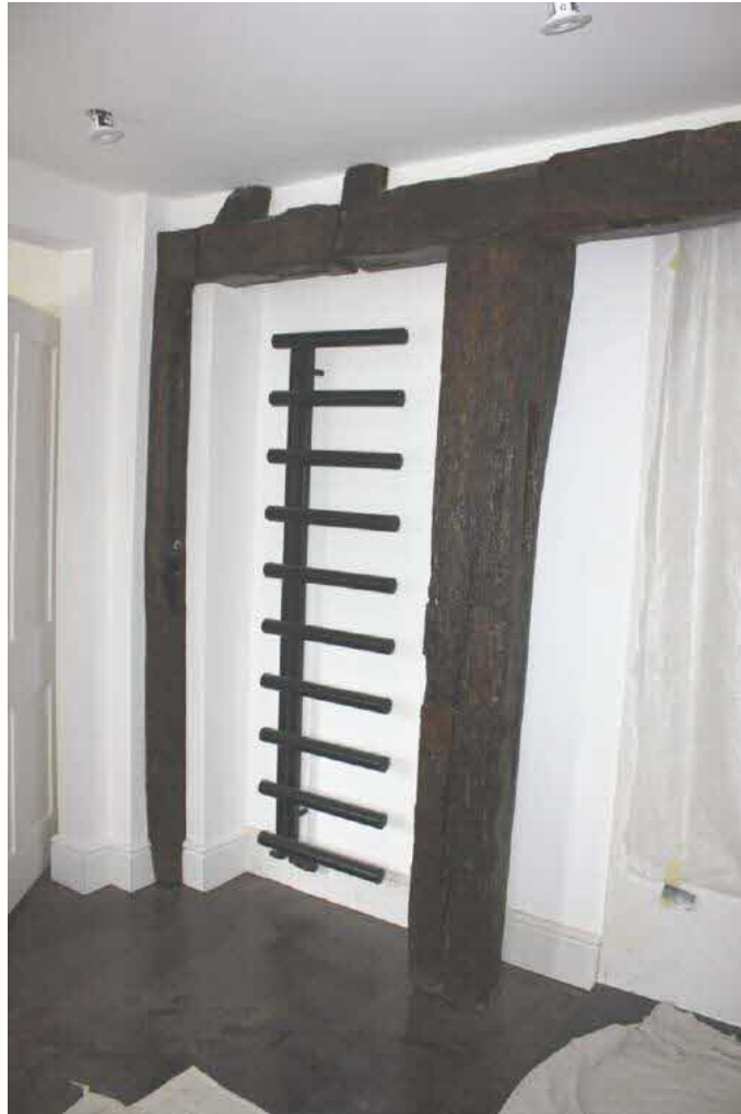
Plate 12. In-situ, pegged framing in the first floor bathroom.
