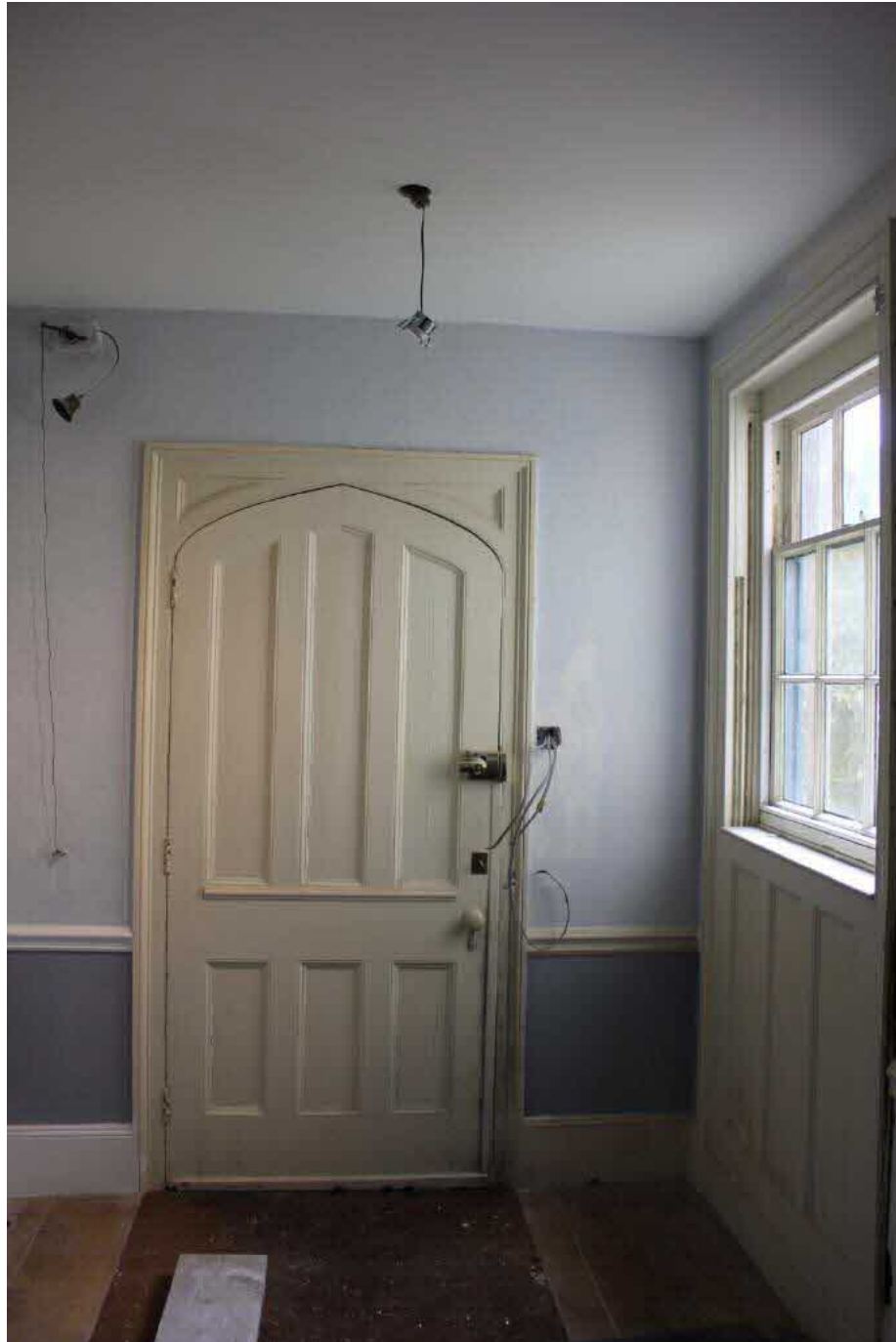
Plate 31. The main entrance door in the lobby.
