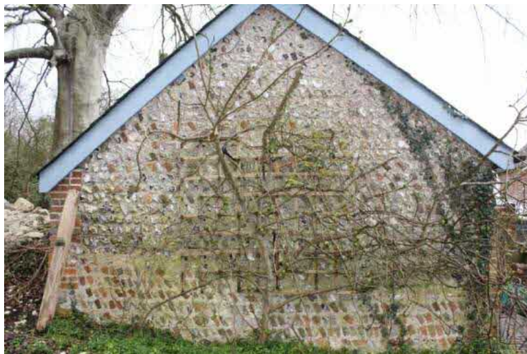
Plate 9. Bungaroosh east wall of the Stable.
