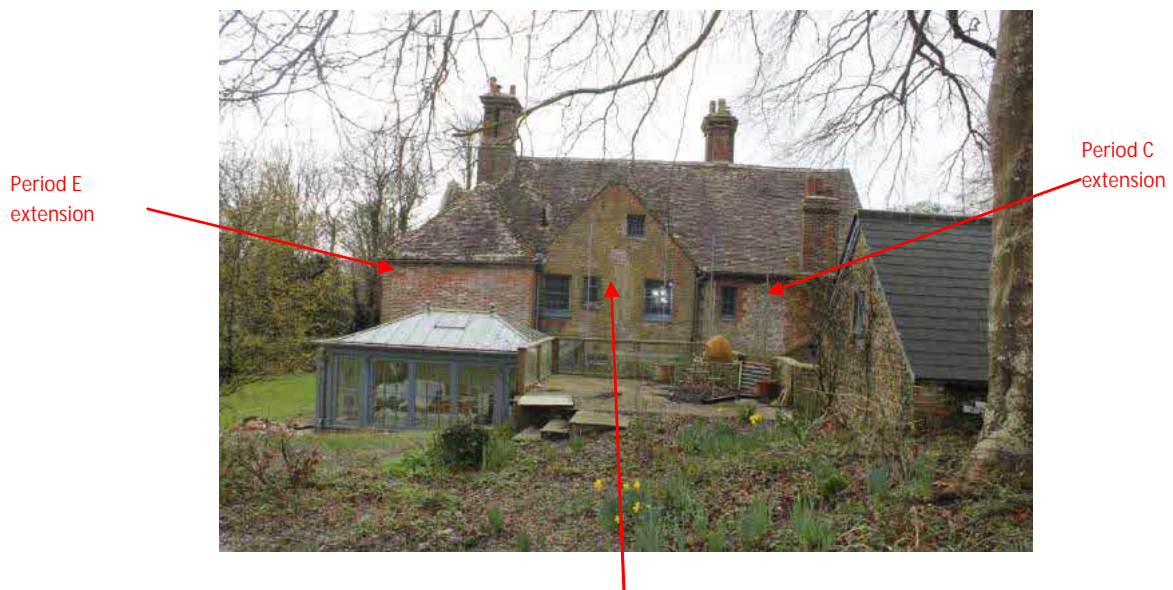
Plate 19. Slightly projecting, central dormer Period D extension to the rear.
