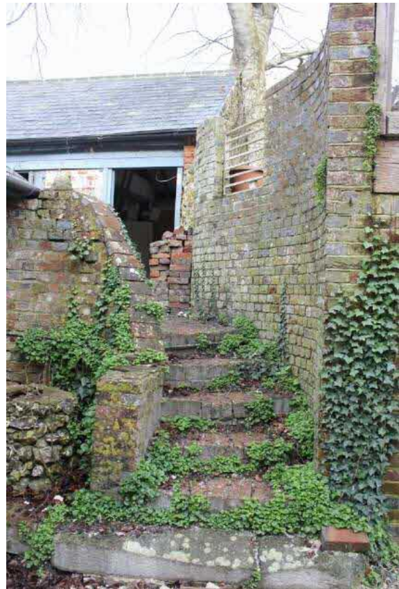
Plate 2. The steps the re-built outbuilding.
