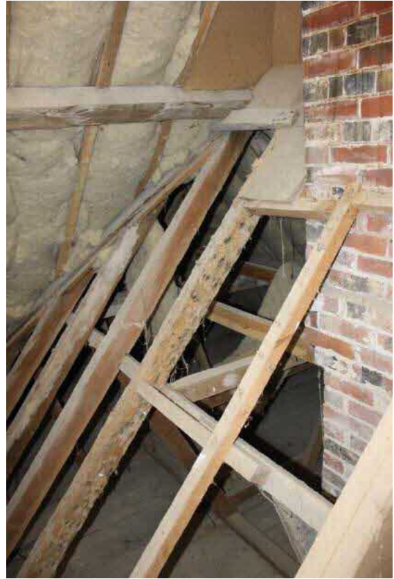
Plate 36. Re-used rafter in the later roof.
