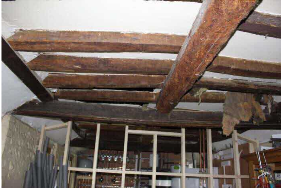
Plate 8. The roof construction of the outbuilding.
