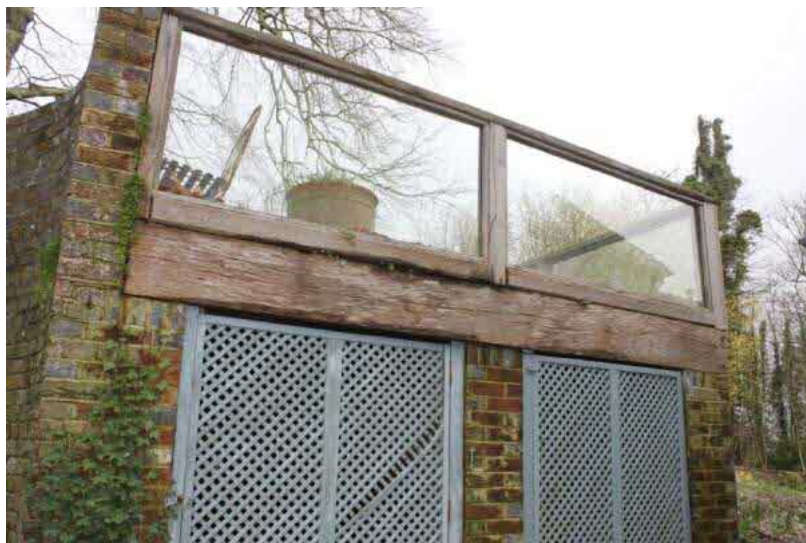
Plate 11. The re-built outbuilding north of the courtyard.
