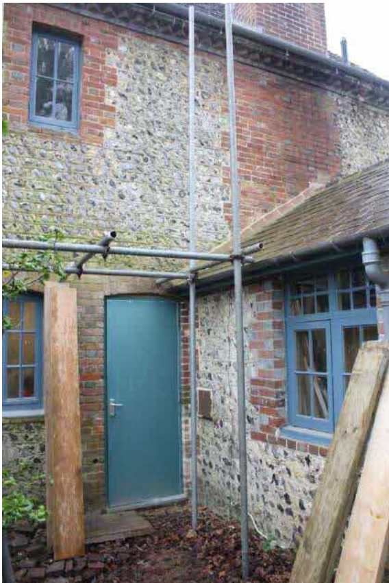
Plate 1. The attached outbuilding
