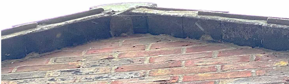
Tightly sealed gable apex at east side of bungalow roof
