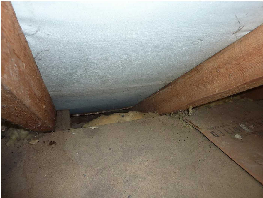
View of eaves from side loft
