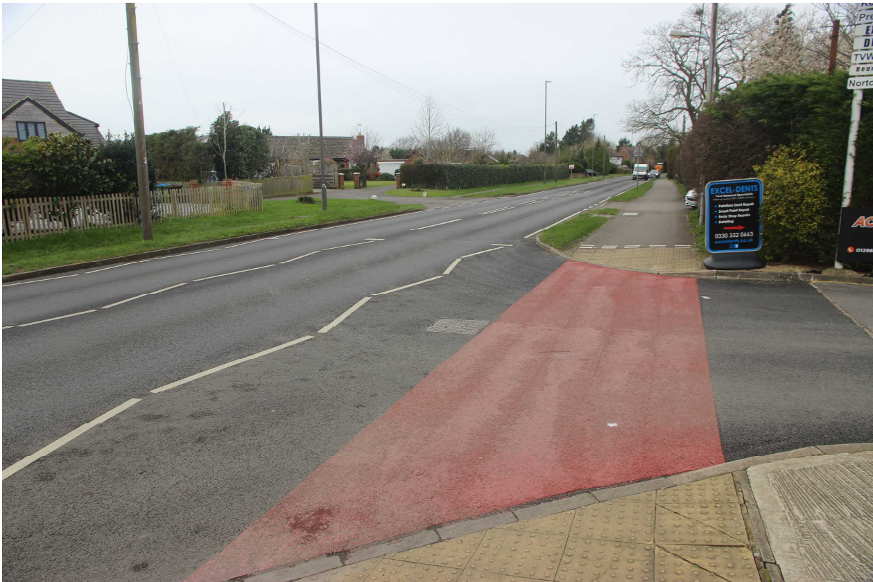
Road adjacent to the access on the SE side of the access towards Aylesbury.
