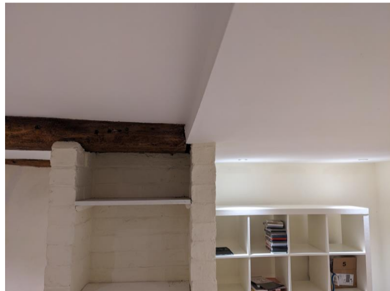
Image 10 Side view of brick pier showing ceiling height differential between Playroom & Extension
