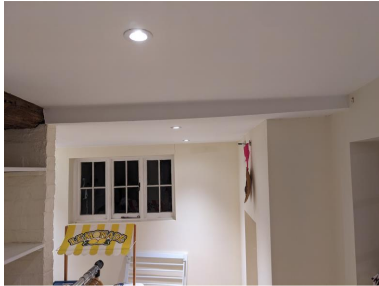
Image 12 View to right of brick pier showing Extension
