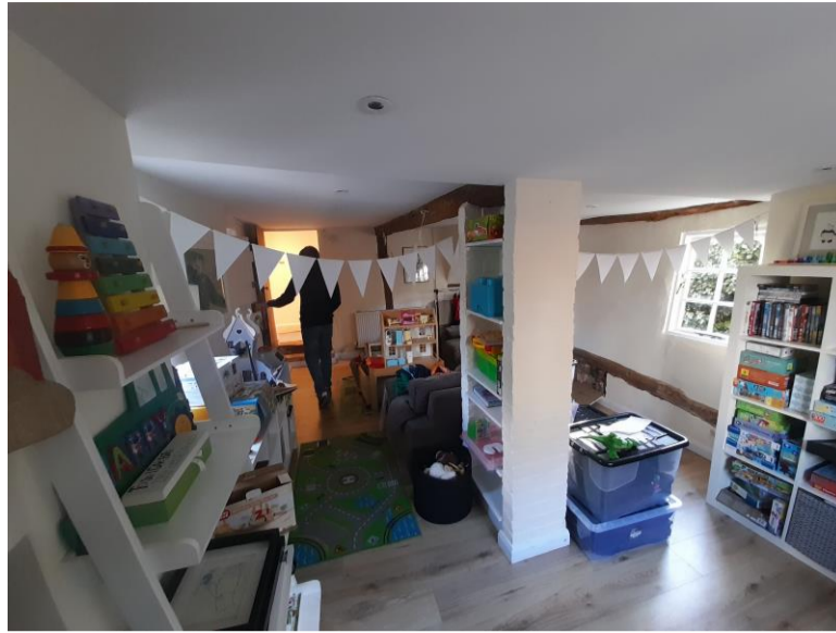
Image 9 View of side of brick pier from extension highlighting awkward space
