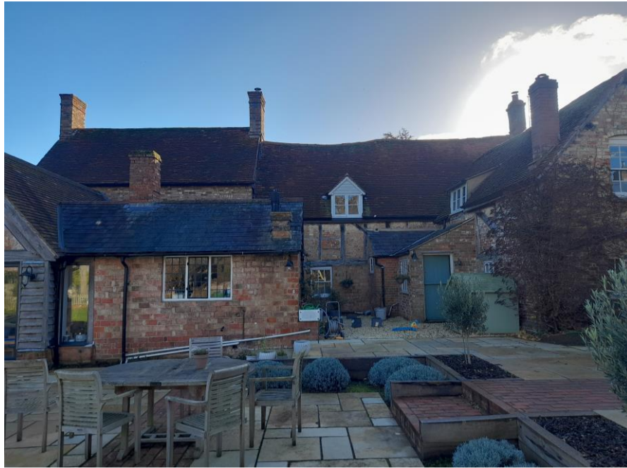
Image 15 Rear elevation of Mill Hook Farmhouse
