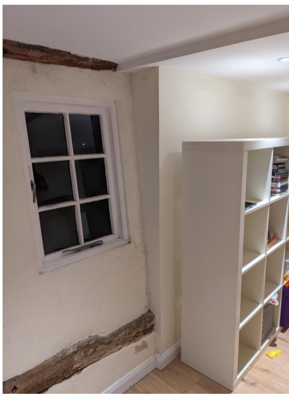
Image 13 Location of new pier to internal face of front wall
