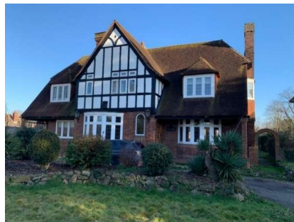
Photograph: Front elevation
