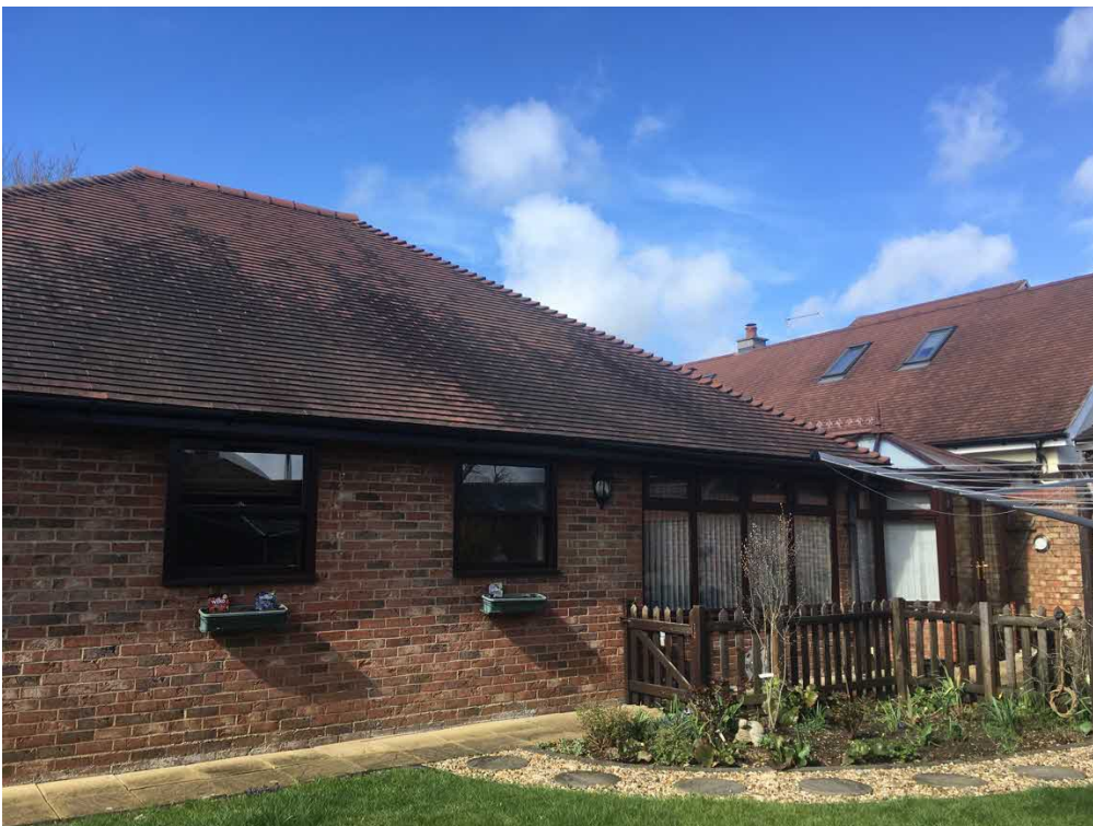
View at Point C: - Existing Side Elevation:
