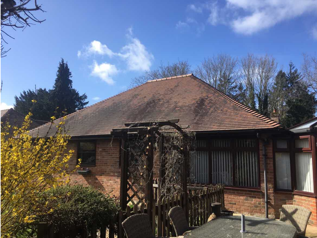
View at Point D: - Existing Side Elevation:
