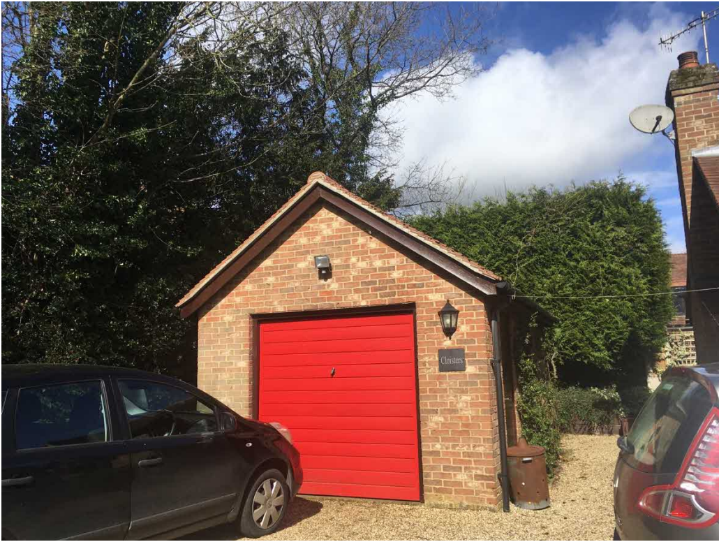
View at Point B: - Existing Garage:
