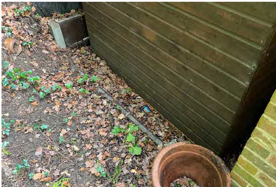
Photographic plate showing existing garden shed, concrete base, and concrete retaining wall to rear of existing building(ROAVR, 2024)
