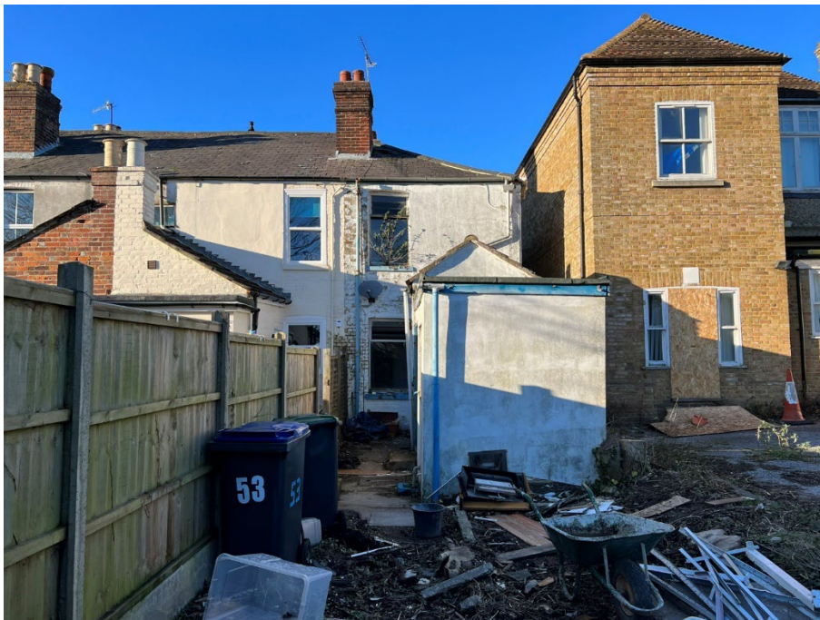
Figure 6 - Photograph from rear garden (nos. 57, 55, 53 & Cossington House Surgery) Jan '24.
