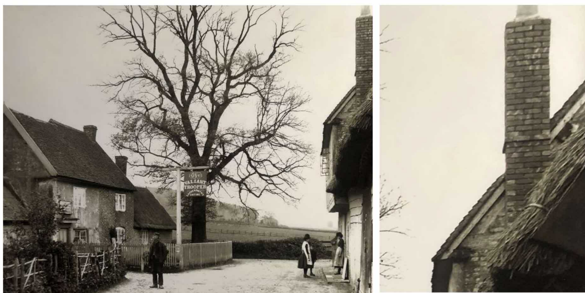
Figure 2: Left - photograph of the northeast gable of 42-44 Trooper Road, the thatched barns (now 40 Trooper Road) and the Valiant Trooper (photograph circa 1900). Right – close-up of the northeast gable where exposed brick and timbers can be observed.
