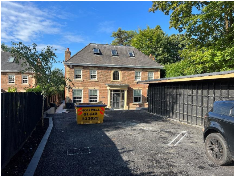
80mm Permeable Tarmac Binder Base Coat 14-20mm open texture
