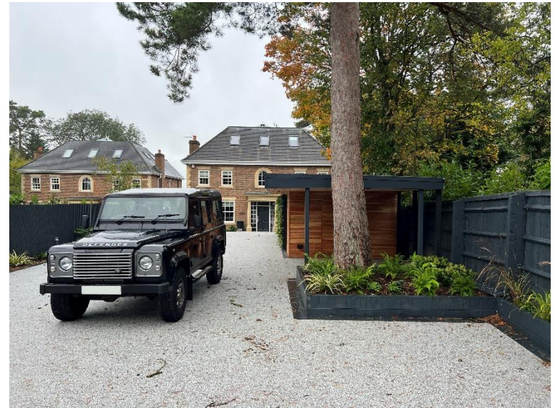
18mm Permeable Resin Bound Surface Course 14-20mm open texture
