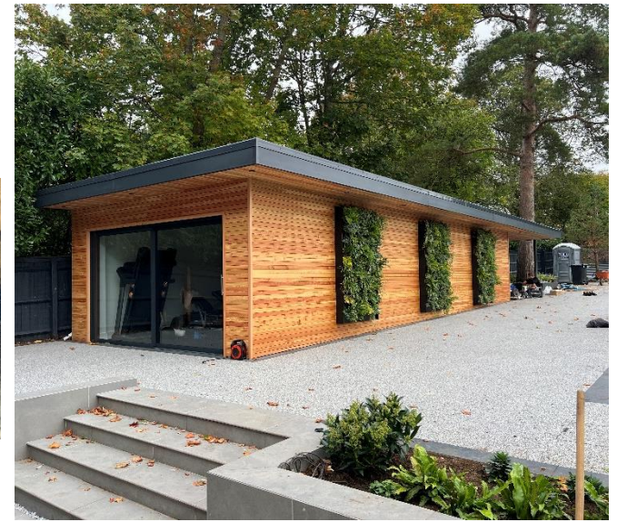
Slimmer outbuilding with timber rainscreen and green walling Permeable resin stone wearing course.
