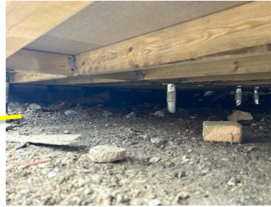
Mini Screw Piles below lightweight shed
