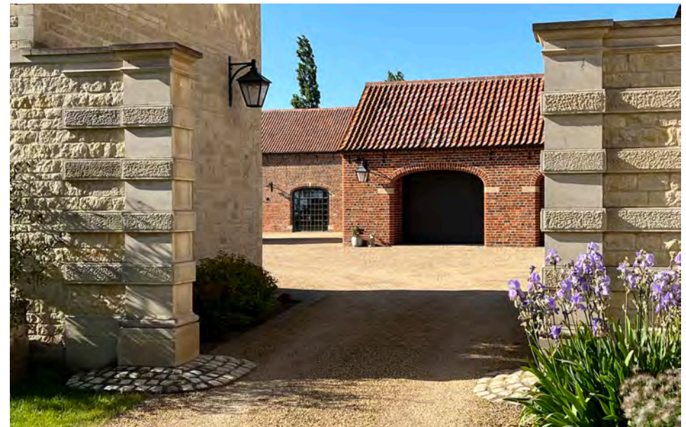
'Tar and Chip' gravel shown here elsewhere on site in already completed areas
