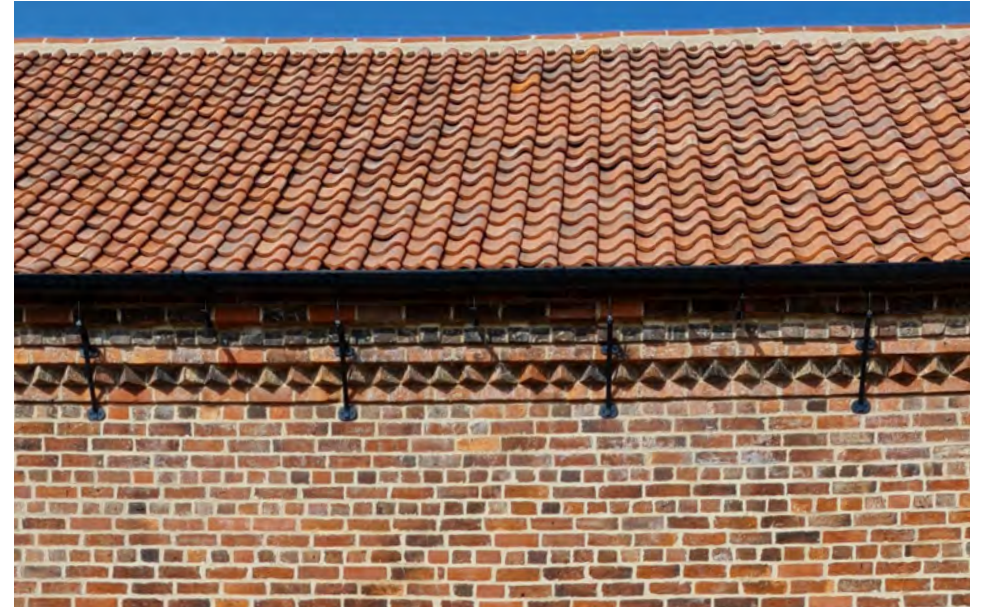
North West Barn - the existing eaves with diagonally set corbelling
