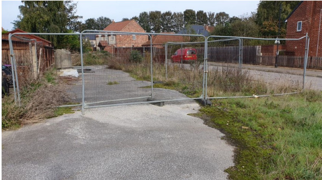
Photograph 1. View of the Site looking north, showing the extent of remaining unvegetated made ground.
