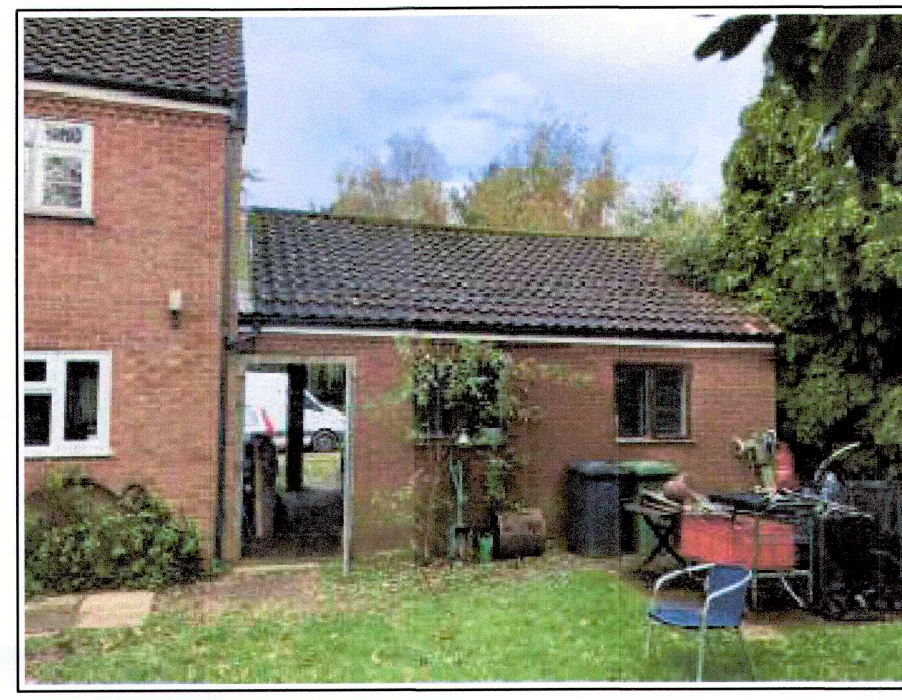
EXISTING CAR PORT (REAR)
