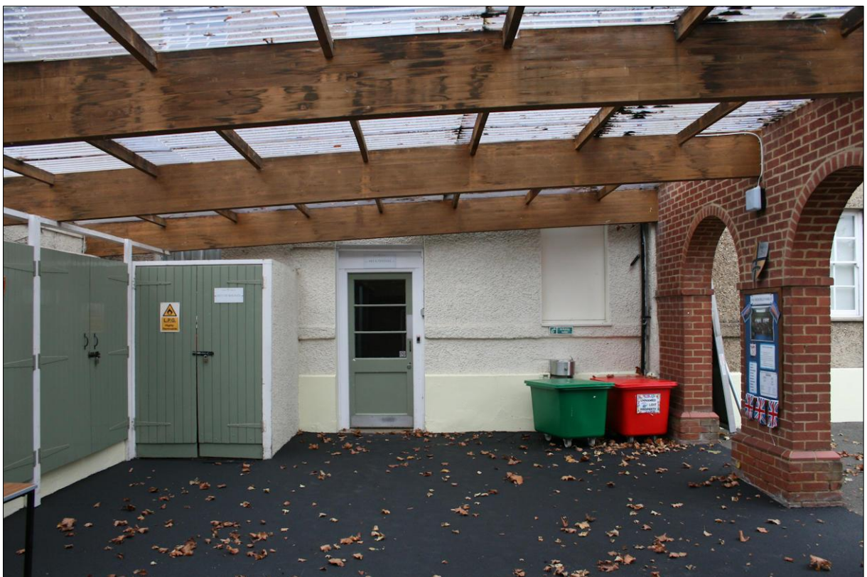
Plate 2: South elevation, west end, from south
