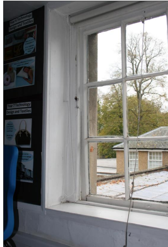
Plate 17: F3 textiles room, detail of south-facing window
