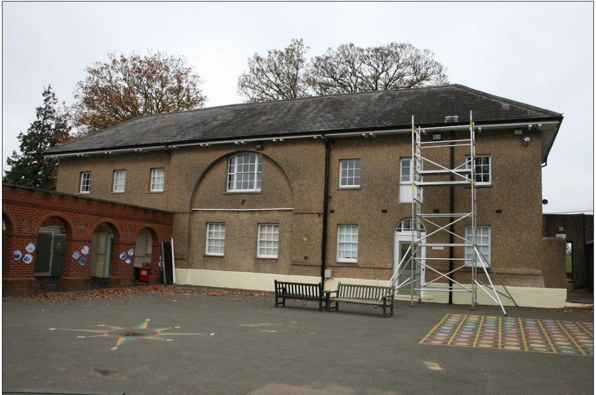
Plate 1: South elevation from south
