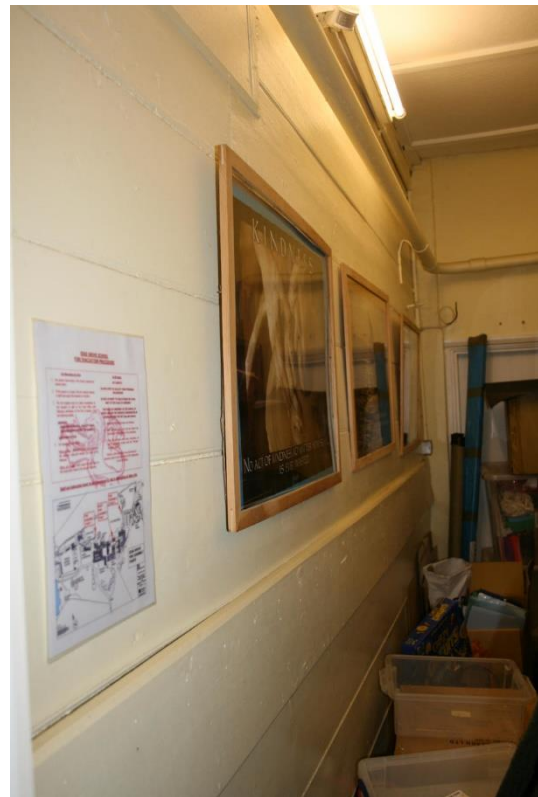
Plate 13: G11 store, timber-clad south wall from east
