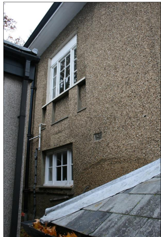
Plate 5: West elevation from south-west
