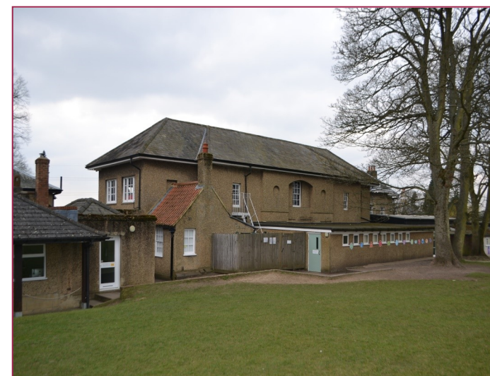
Rear elevation of Stable Block
