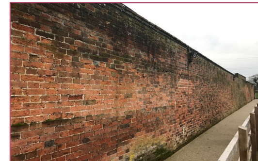
Refurbished northern wall to the Walled Garden
