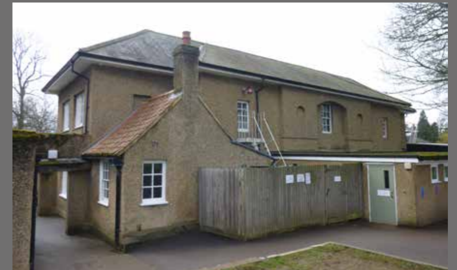
Existing North East Corner
