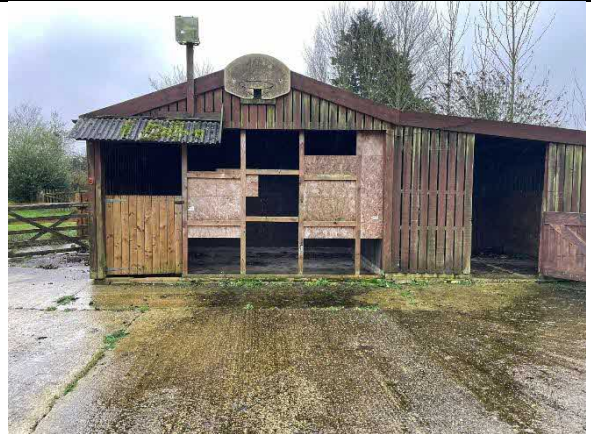
Photo 14 – North gable elevation
