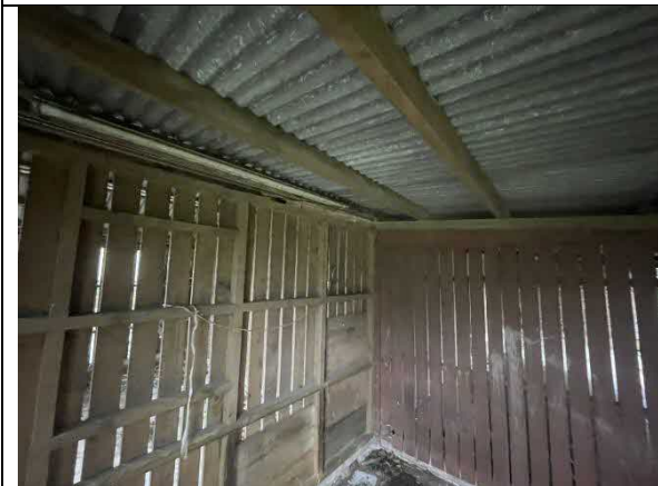
Photo 21 – Internal view of the lean-to
