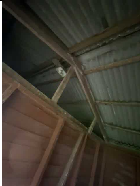
Photo 20 – Internal roof view showing timber purlins supporting corrugated sheeting off an internal loadbearing wall
