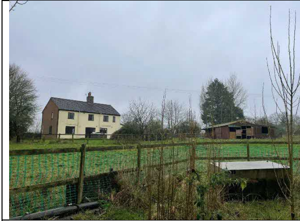
Photo 1 – View of the property from the north with the outbuilding visible to the right
