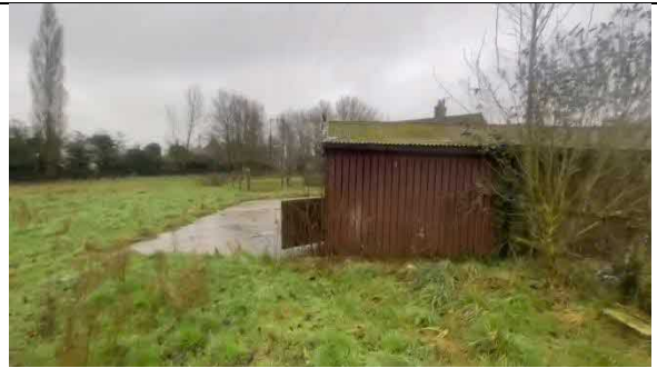
Photo 16 – West elevation detail
