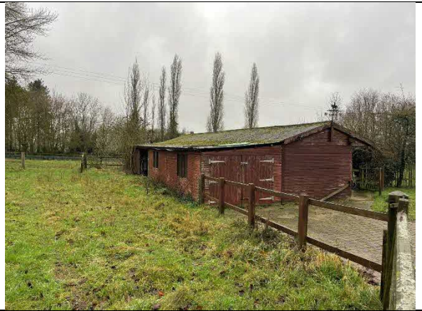
Photo 4 – General view from the south-west
