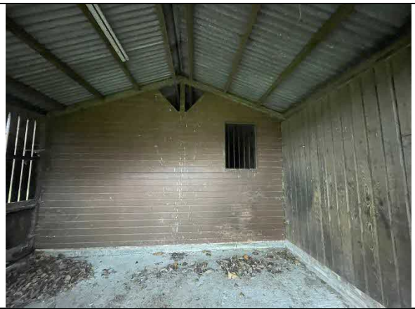
Photo 18 – Internal view at the northern end
