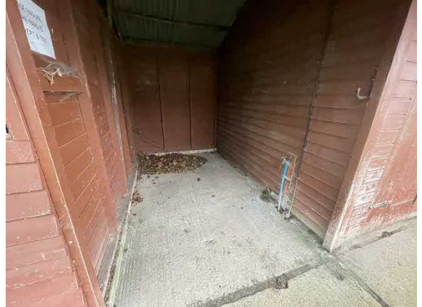
Photo 10 – Recess on the east flank
