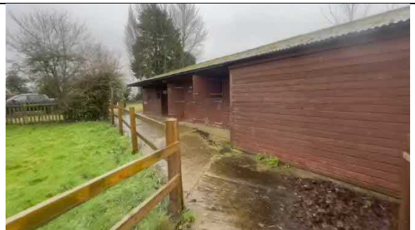
Photo 12 - View of the east flank wall from the north-east
