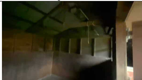
Photo 20 – Internal roof view showing timber purlins supporting corrugated sheeting off an internal loadbearing wall
