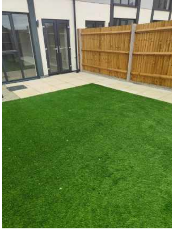
One of the plots with the artificial grass installation complete.
