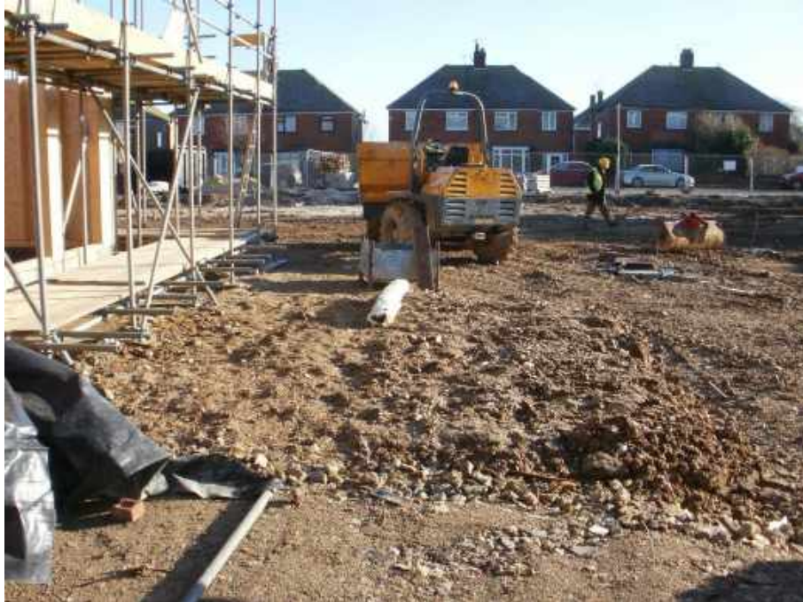
Looking east across the centre of the southeast area of the site showing the natural ground (head deposits) at the location of the proposed gardens to plots 12 to 14.
