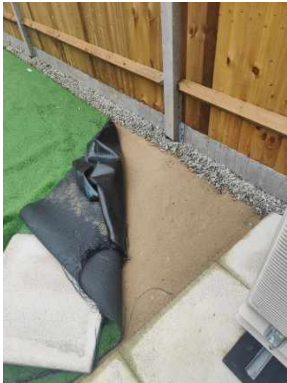
One of the plots showing the sand screed laid for the artificial grass.
