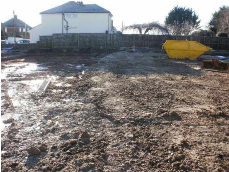
Looking south across the southeast area of the site showing the natural ground (head deposits) at the location of the proposed gardens to plots 15 to 23.
