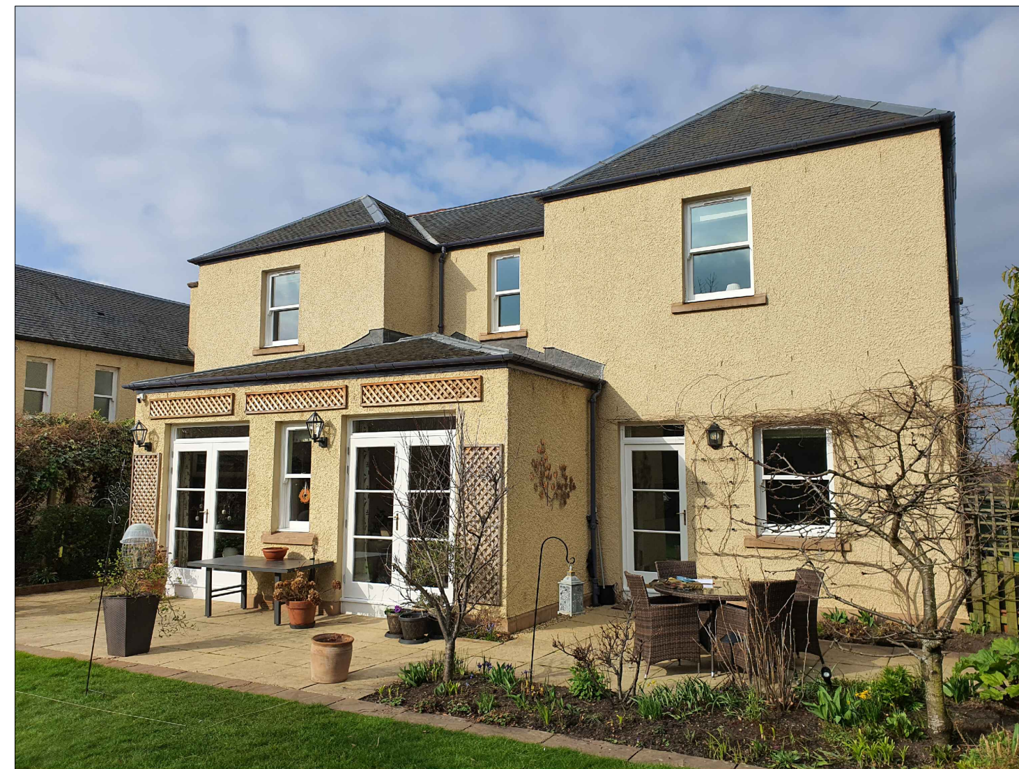
PHOTO TOWARDS ELEVATION 1 1:100
