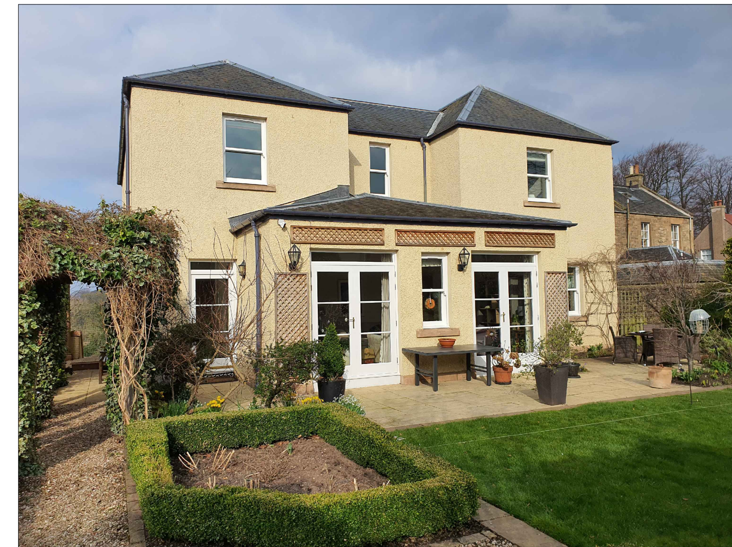
PHOTO TOWARDS ELEVATION 1 1:100
